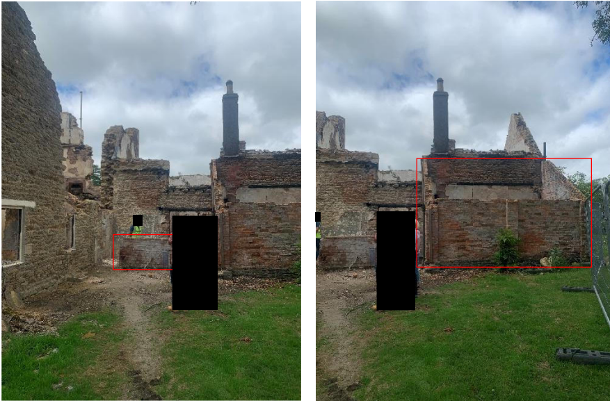
Figs. 02-03. Remains of modern lean-to extensions built from brickwork (marked in red). Photo taken on the 22 nd of July 2024, after approved demolition works have been completed.
