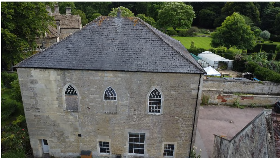
Plate 10 roof area of the hall has some limited potential but no evidence of use
