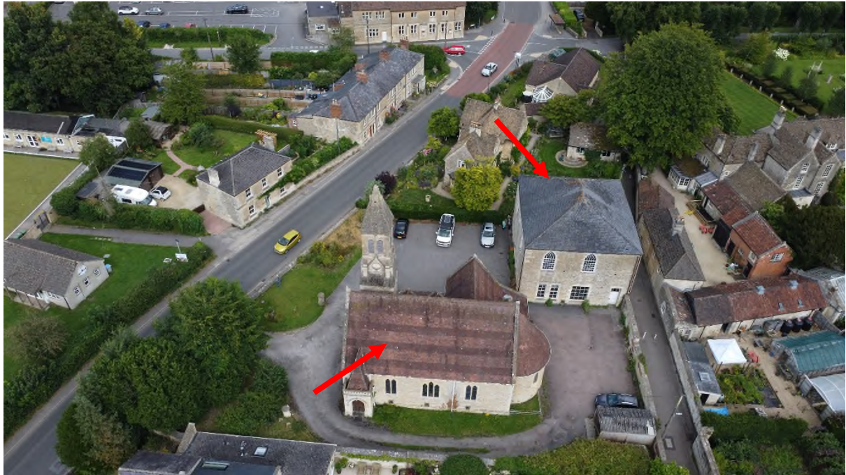
Plate 1 Buildings being surveyed Holt URC church and church hall
