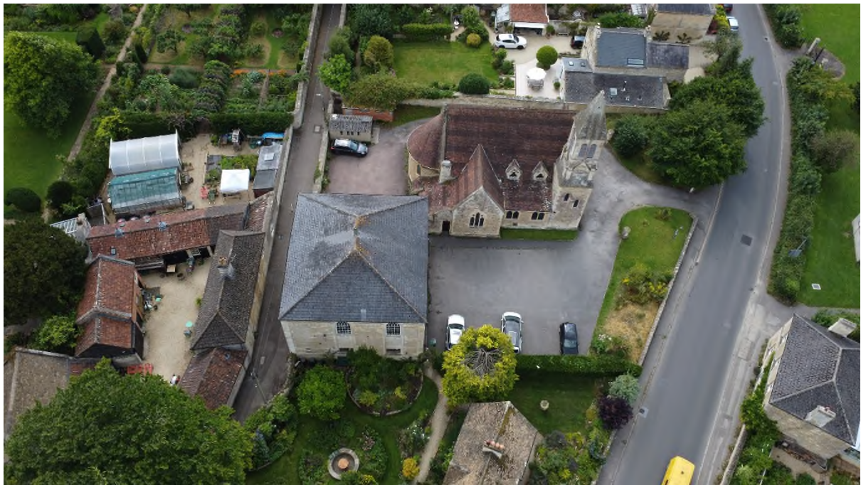
Plate 2 church hall and church looking south west
