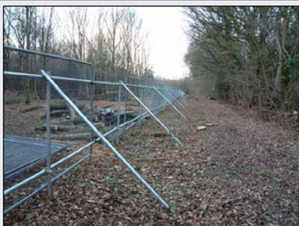
Heras fencing wired to scaffold braced posts
