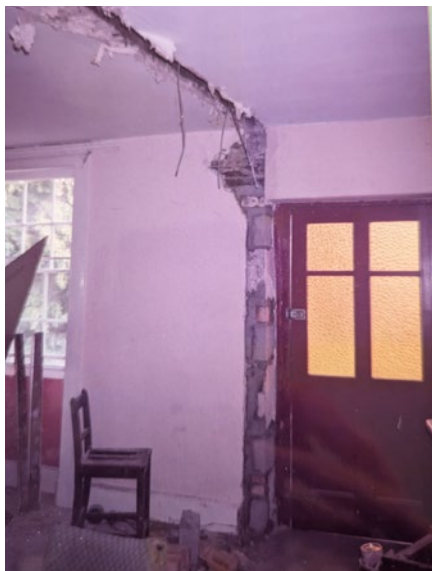
Figure 14 - Partition removed at ground floor
