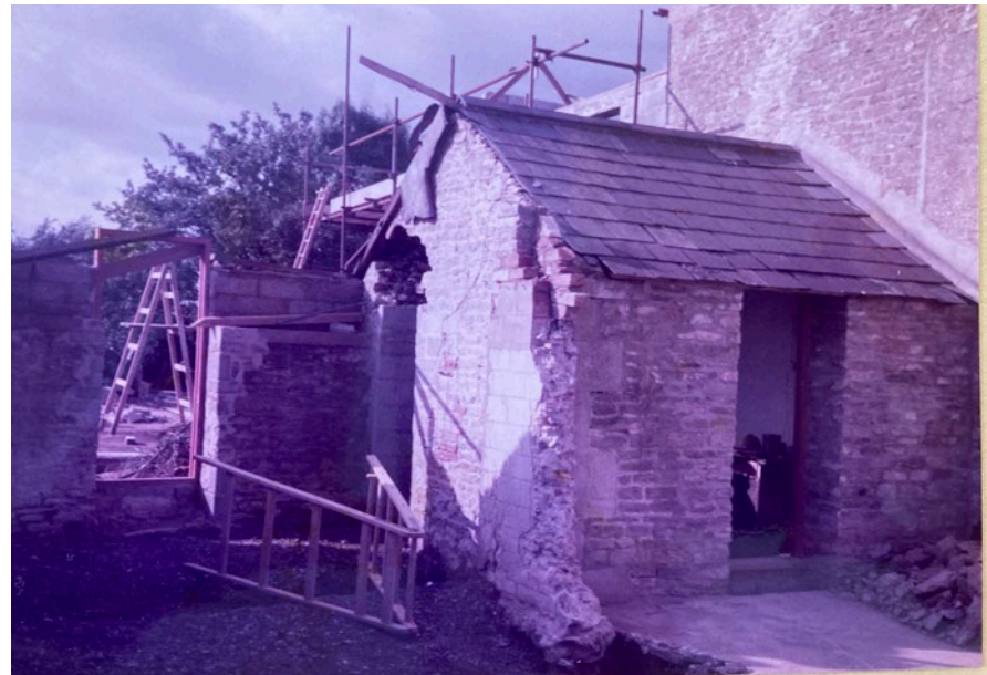
Figure 9 - South east elevation with rebuilt entrance (door and window removed)
