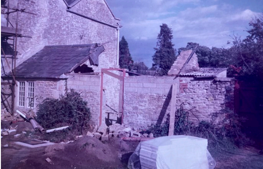
Figure 10 - North west elevation with reused window
