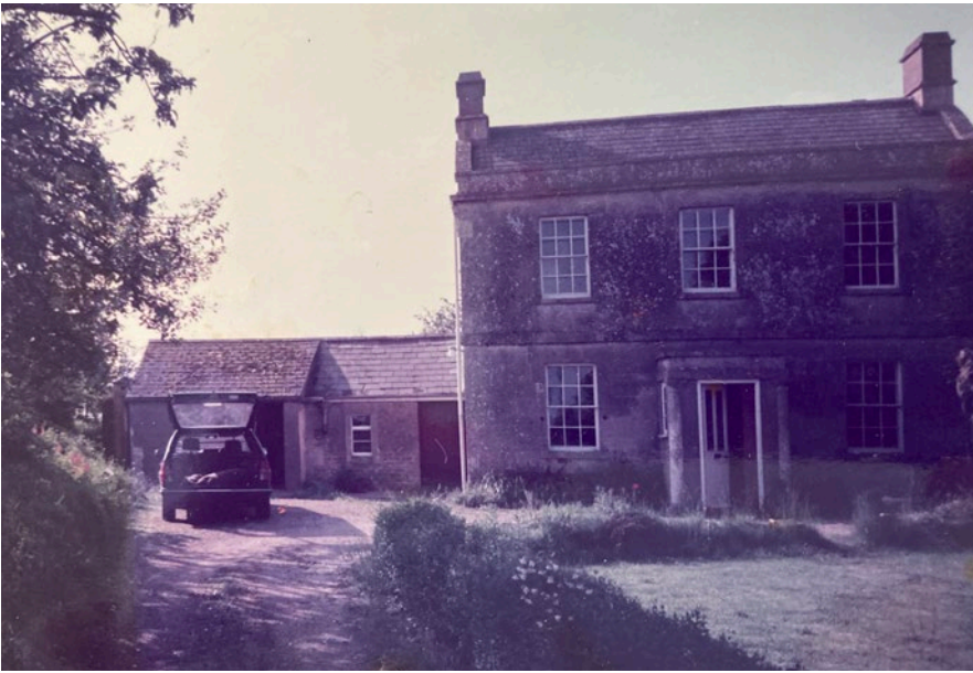
Figure 8 - South east elevation of the south west service range
