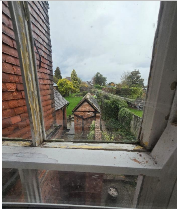
F4 Upper sash bottom rail centre-right
