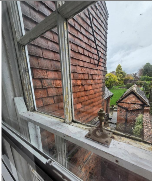
F4 Upper sash bottom rail centre-left
