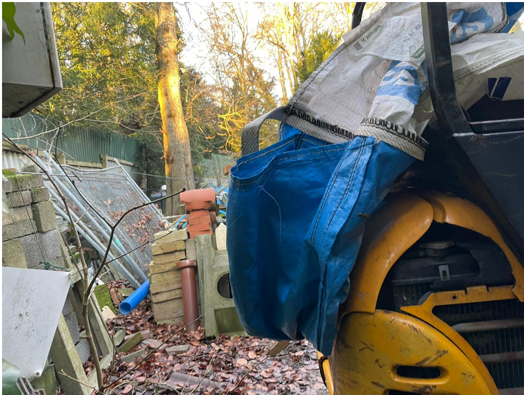
Plant and builders materials stored within the site
