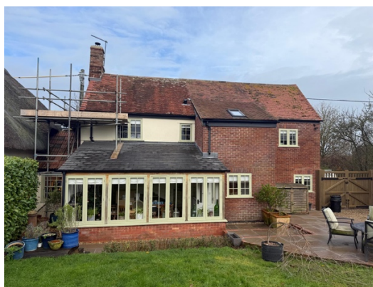
2. The rear elevation and dining room extension
