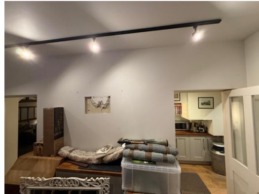
4. Opening up work in dining room
