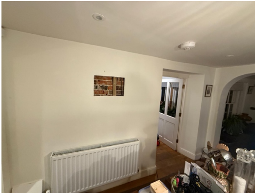
3. Opening up work on kitchen side wall
