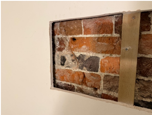
5. The exposed brickwork
