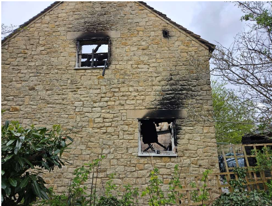
Photo 4 – East Side Elevation – Post Fire
