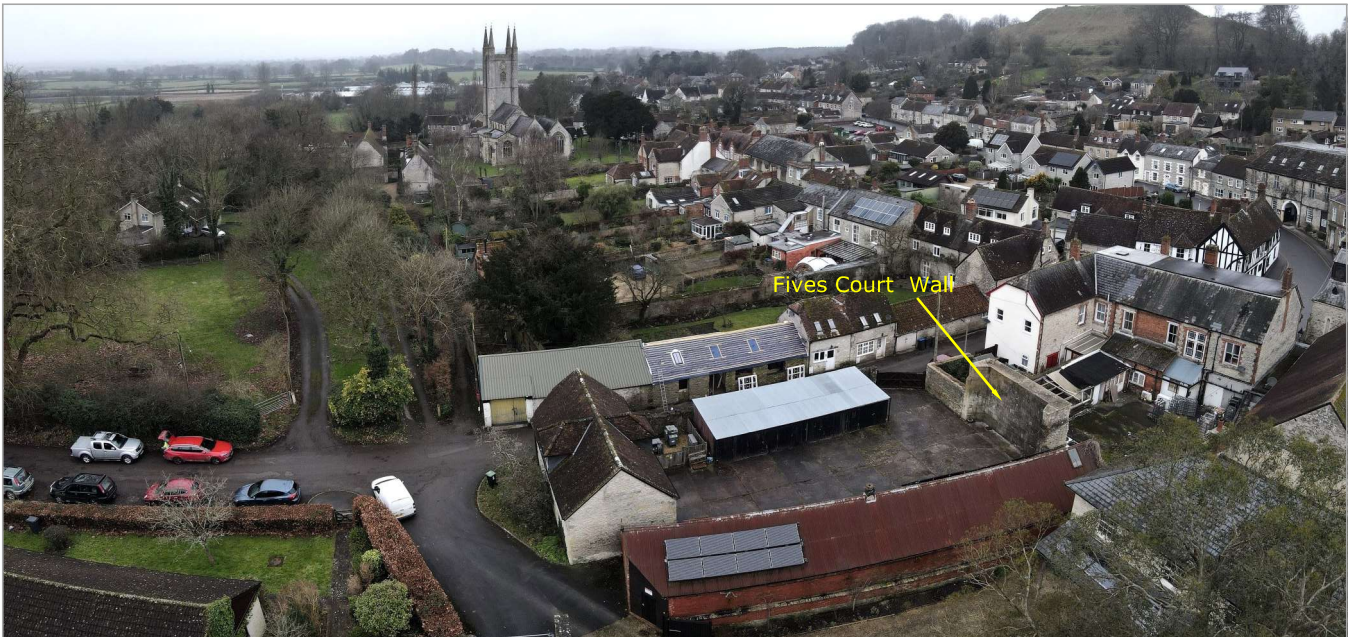
6. Aerial view taken from directly above the site, looking west and north-west. The so-called Fives Court Wall, which is a listed structure, is indicated.
