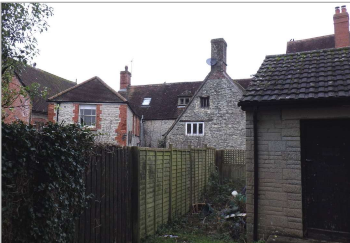
2. View of the rear of nos. 4 and 5 The Square, from inside the site at its northern end. View to north.
