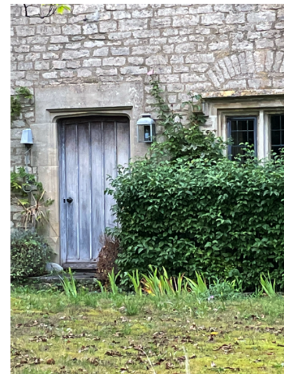
Plank and batten oak front door to Tudor House, listed building in Oaksey
