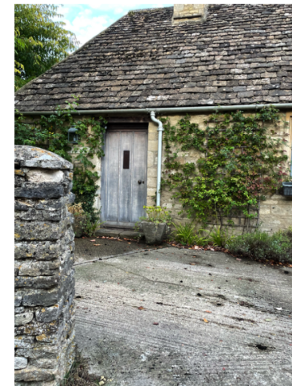
Plank and batten oak side door to Tudor House, listed building in Oaksey
