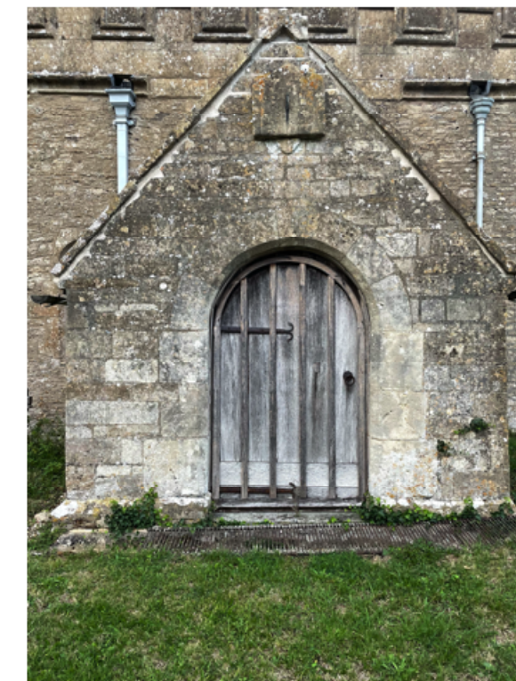
Plank and batten oak rear door to the Church of All Saints, listed building in Oaksey
