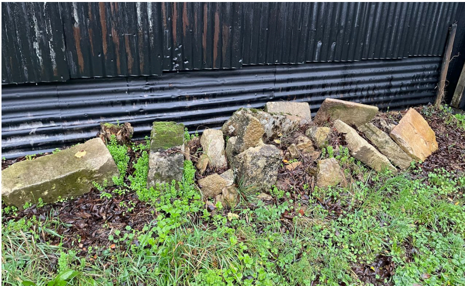
Figure 2: Existing stone on site to be reclaimed for extension cladding (photo client)
