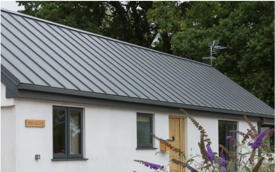
Figure 3: Example of Catnic coated steel roof (catnic.com)
