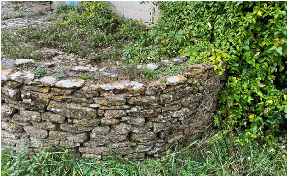
Figure 1: Existing stone on site to be reclaimed for extension cladding (photo client)
