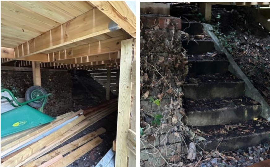
5.5 Above: Historic steps and embankment under decked area.
