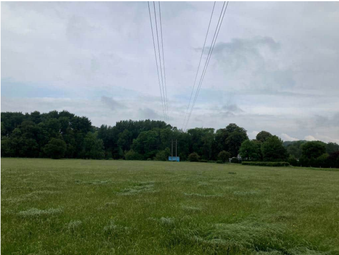
Photograph 6 – View north through the central field along the path of the overheads.
