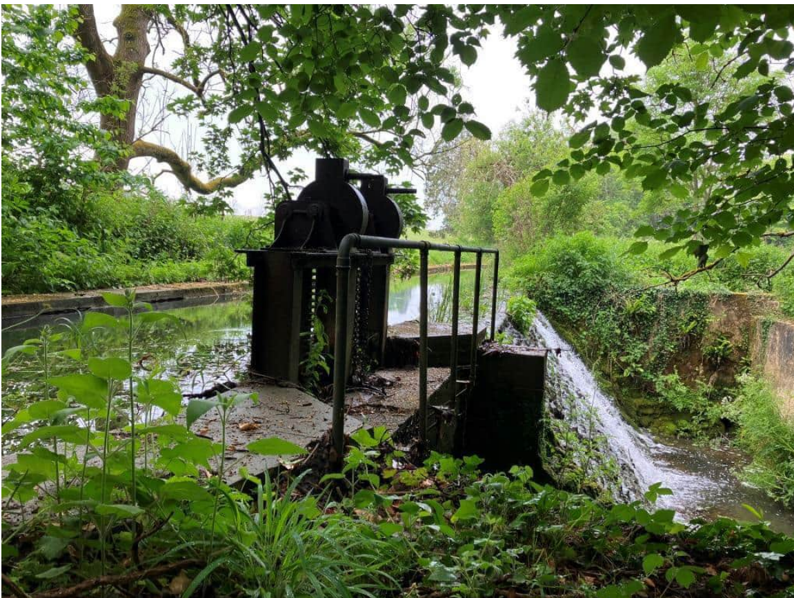
Photograph 14 – Sluice gate and weir associated with Draycot Lake to the northeast of Site.
