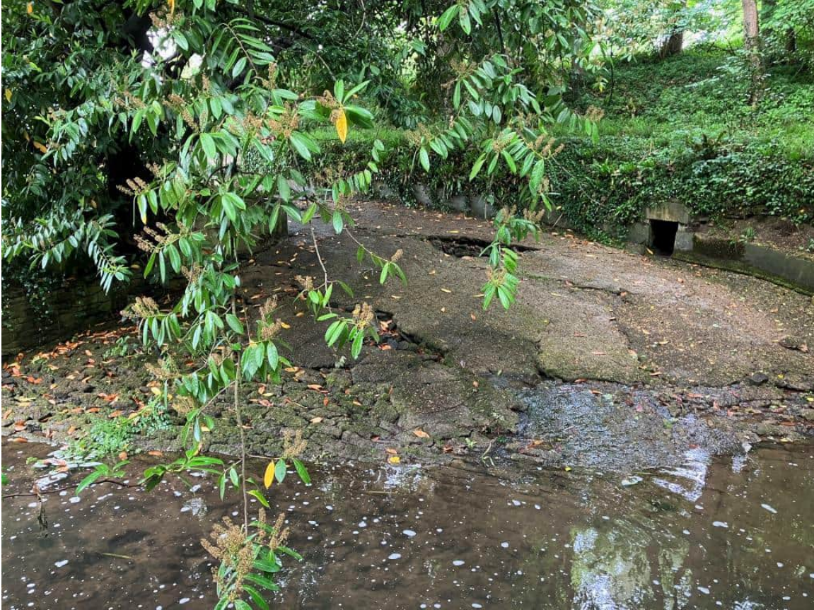
Photograph 15 – Concrete overflow connecting Draycot Lake to the watercourse to the north of Site.
