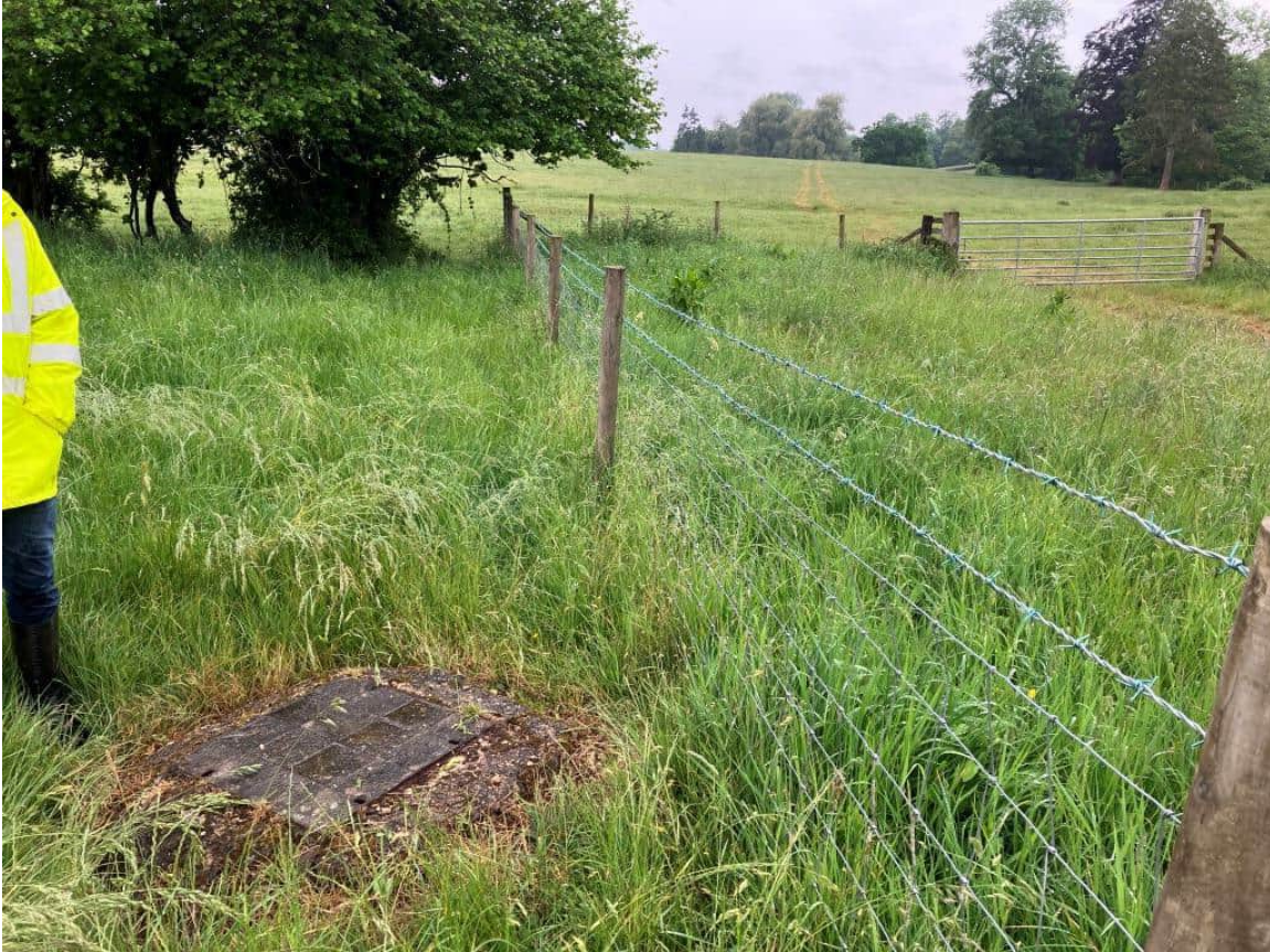
Photograph 7 – Manhole in the northeast corner, associated with foul sewer trending northeast to southwest across Site.
