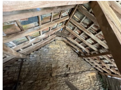
7: Garage section interior.
