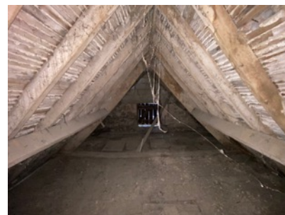
15: Building 7 – roof void.
