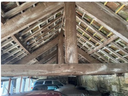
6: Interior – main section.
