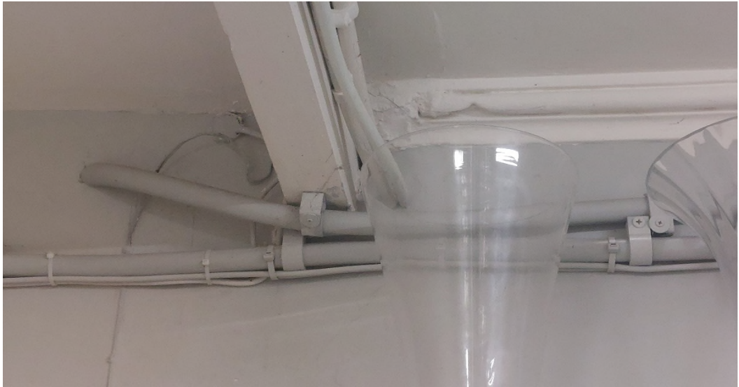
Figure 10 The east wall of the back entrance hall showing the cornice to the southern part of the room which does not continue north of the cross beam to the ceiling.
