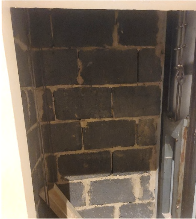
Figure 7 The interior of the shaft of the dumb waiter showing the blockwork of the structure.
