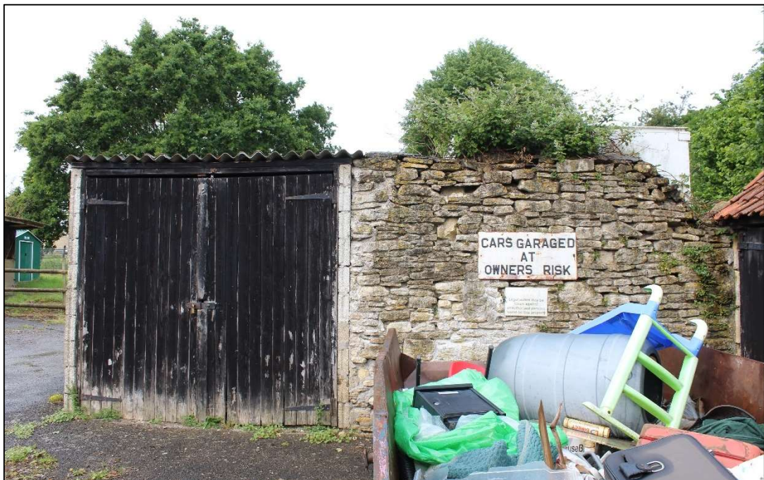
Photo 11 Building D: east elevation
