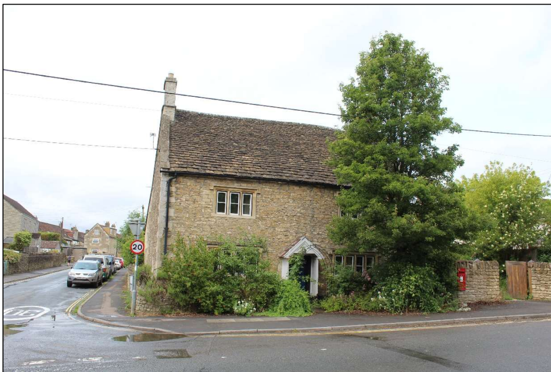
Photo 31 Bath Road Post Office: principal elevation as viewed from Bath Road
