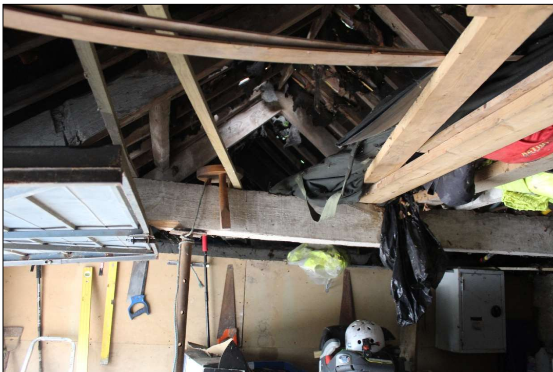
Photo 9 Building C: roof structure
