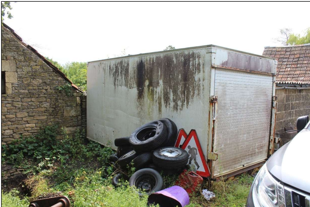
Photo 13 Building E overview, looking south-east
