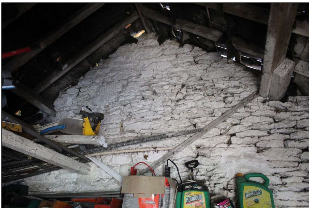
Photo 10 Building C: material detail
