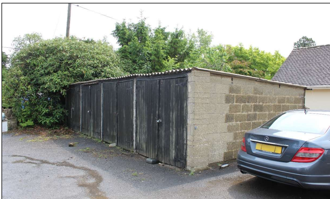
Photo 20 Building N, looking south-east
