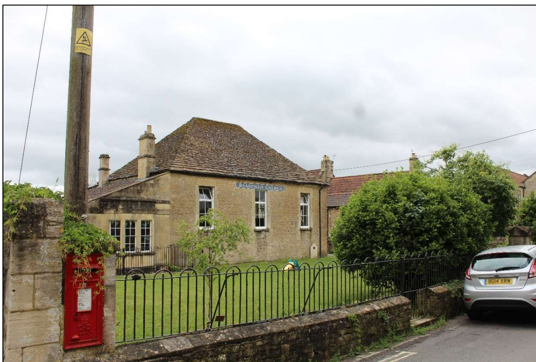
Photo 24 Bearfield Congregational Chapel, looking south-east
