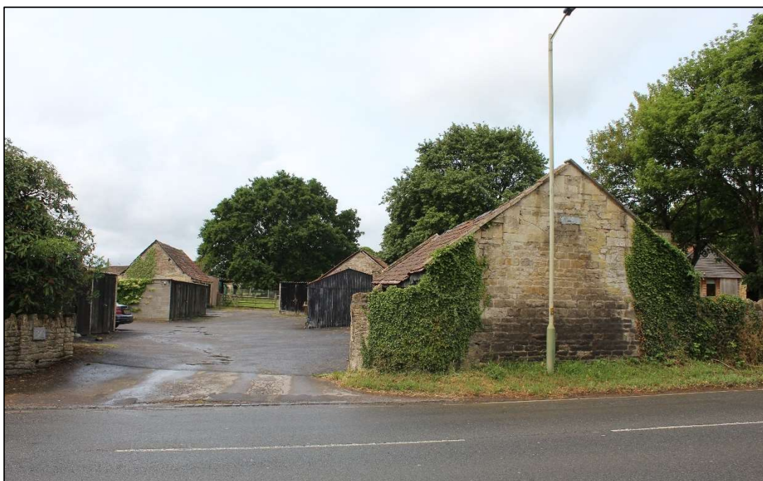
Photo 1 Overview of the Site from Bath Road, looking west
