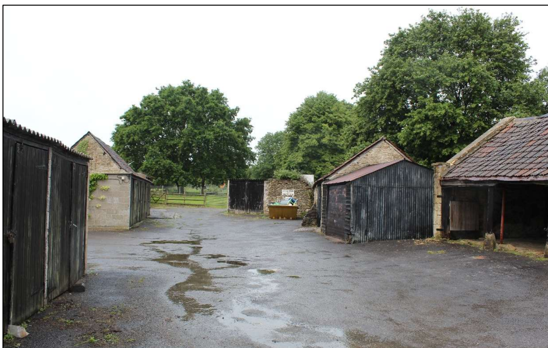
Photo 2 View into the Site, looking west
