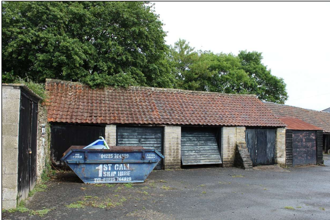
Photo 8 Building C: south elevation
