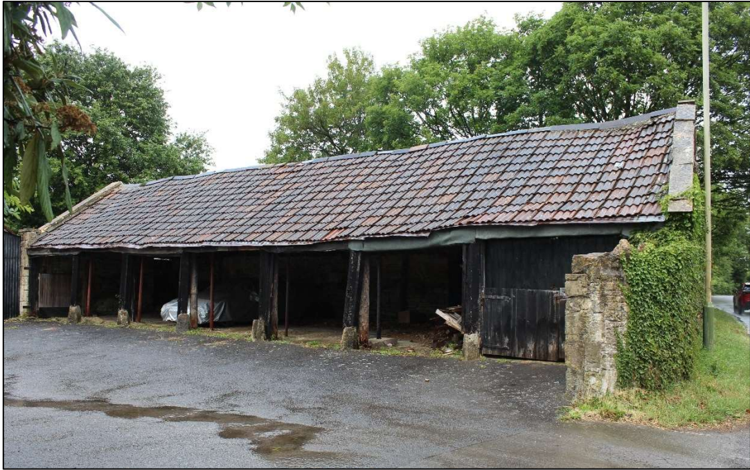
Photo 3 Building A: south-east elevation
