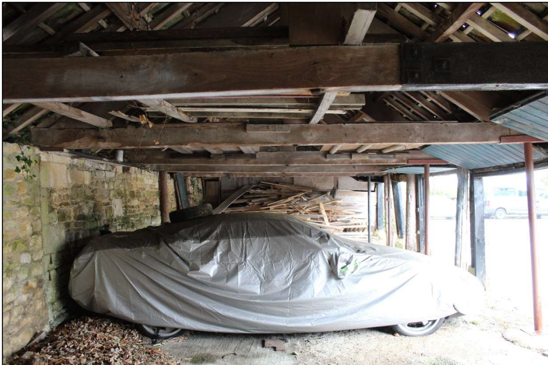
Photo 5 Building A: interior view, looking north-east
