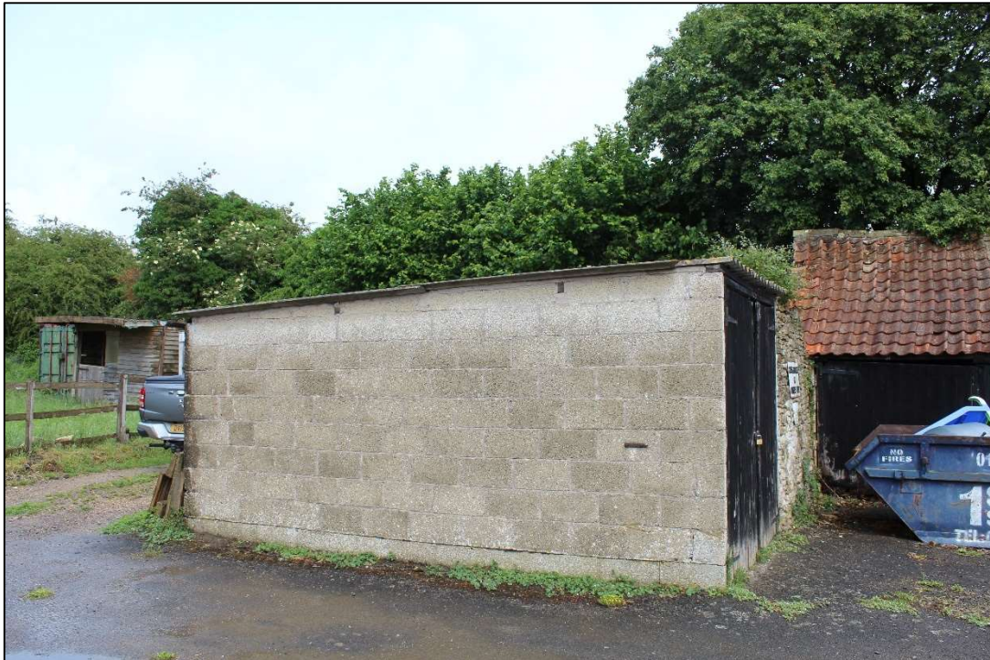
Photo 12 Building D: south elevation
