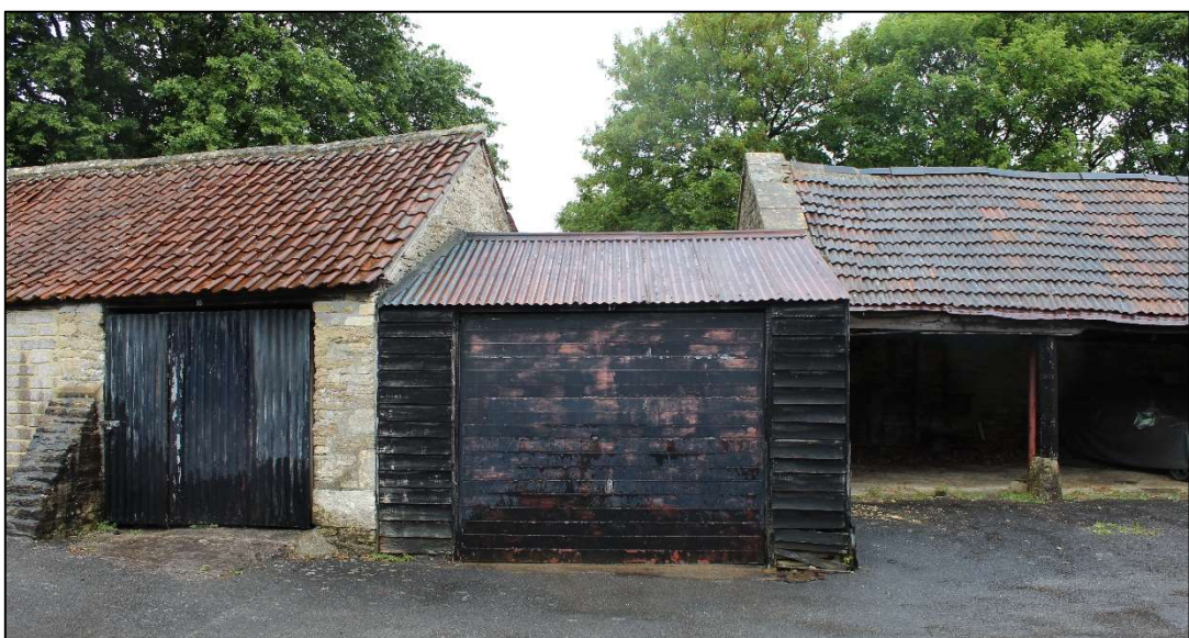
Photo 7 Building B: South-west elevation
