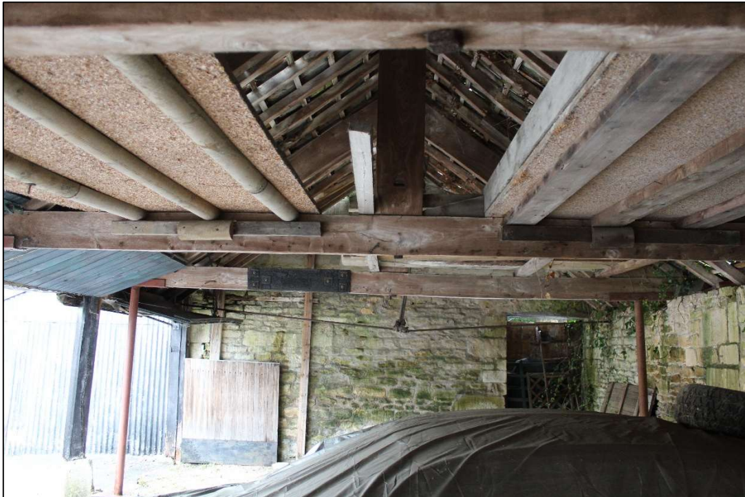
Photo 6 Building A: interior view, looking south-west
