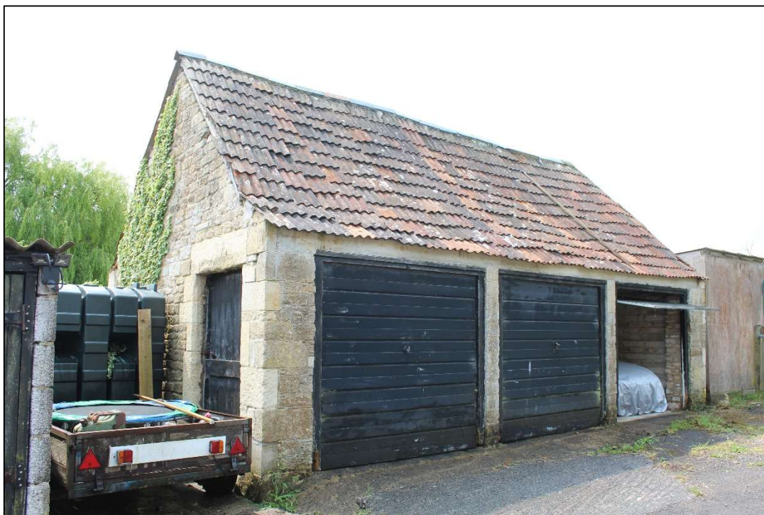
Photo 16 Building L: north-west (principal) and north-east elevations
