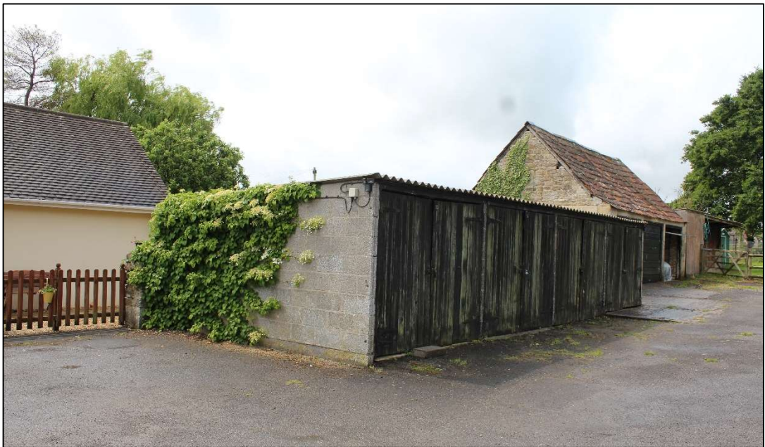
Photo 19 Building M, looking south-west
