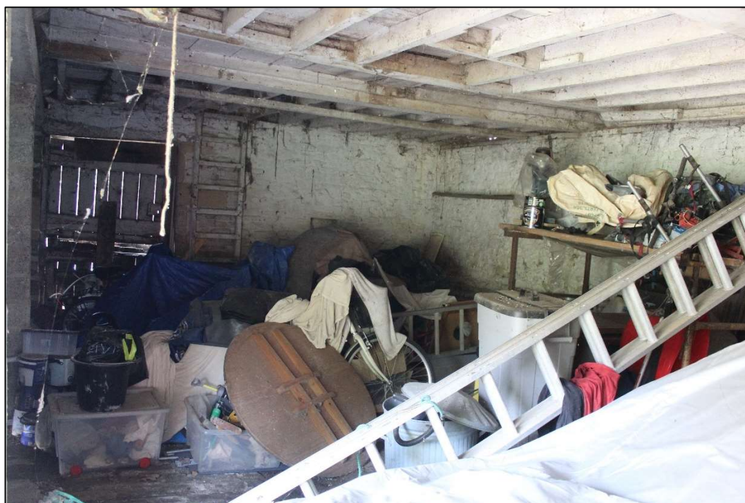
Photo 18 Building L: interior view looking north-east
