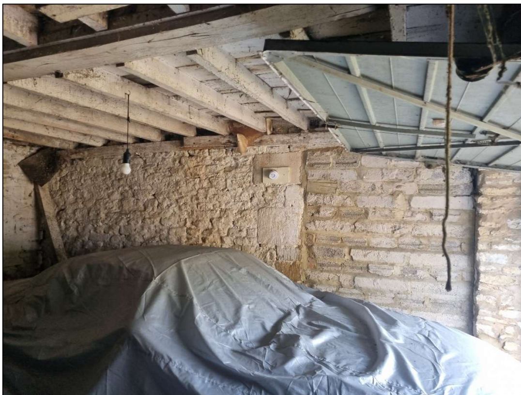
Photo 7 Building L: interior view looking south-west, showing blocked opening
