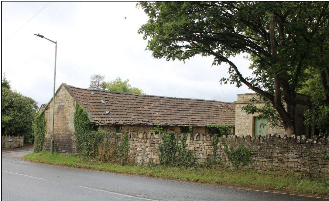
Photo 4 Building A: north-east and north-west elevations of Building A, as viewed from Bath Road
