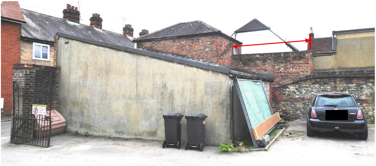
Photographs indicating section of wall to be demolished and rebuilt
