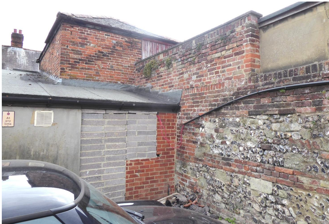
Fig 2.1: East end of north boundary to 35 Rollestone Street with attached shed
