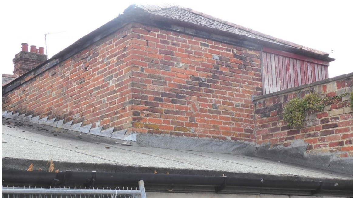
Fig 3.3.1: Boundary wall abutment to the two storey block
