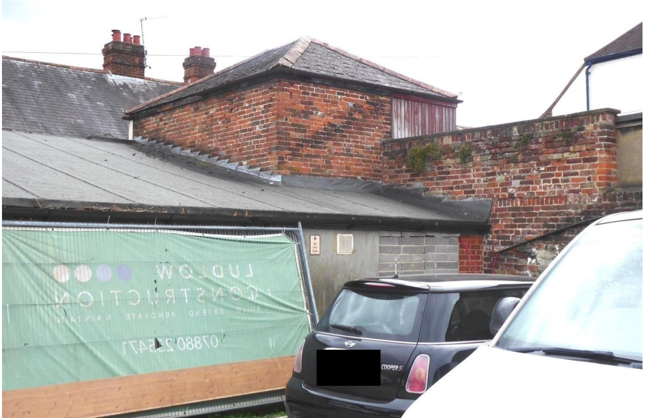
Fig: Boundary wall abutment to two storey section from the northwest
