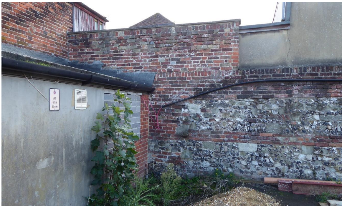
Fig 7.1.4: Varied build phases to north boundary wall
