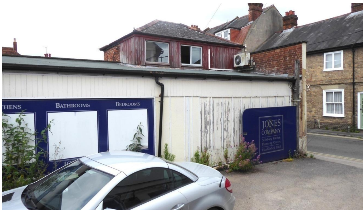
Fig 2.2.2: Single storey building against the north boundary wall
