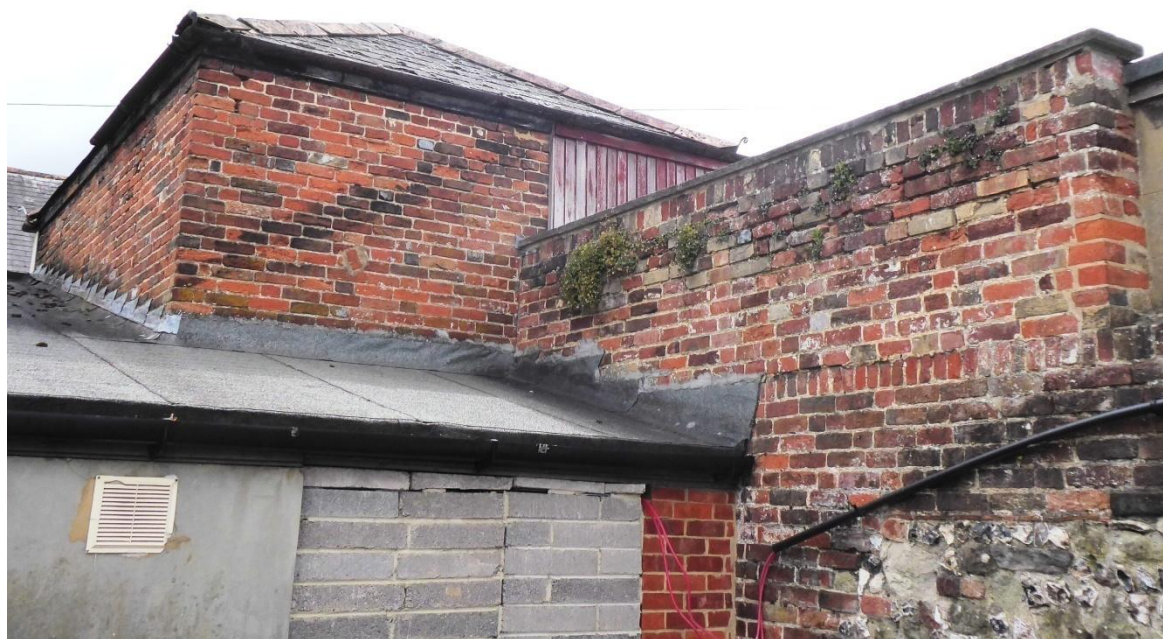
Fig 3.3.9: North boundary wall abutment to two storey block from west
