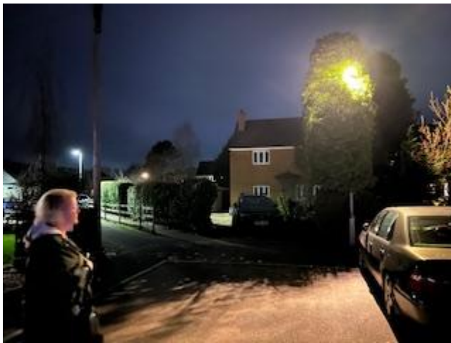
Photo 10: Electric pole at night, ivy obscuring the light
