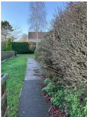
Photo 8 Hedge encroaching footpath at barrier end
