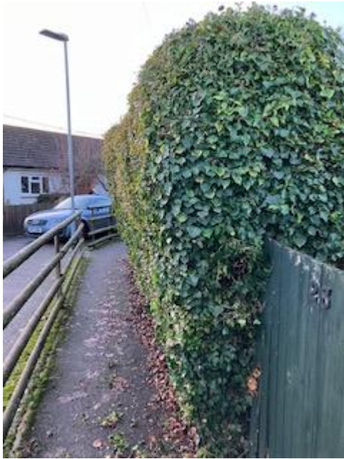
Photo 7 Hedge encroaching footpath from gate
