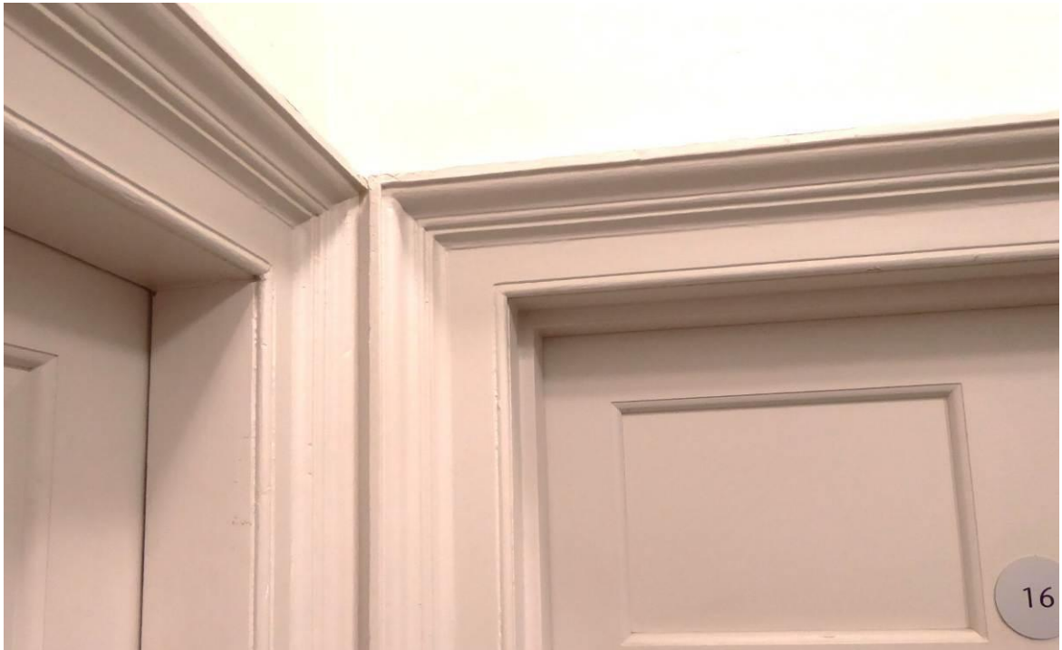
Fig 3.1.1: Original pattern door linings and architraves
