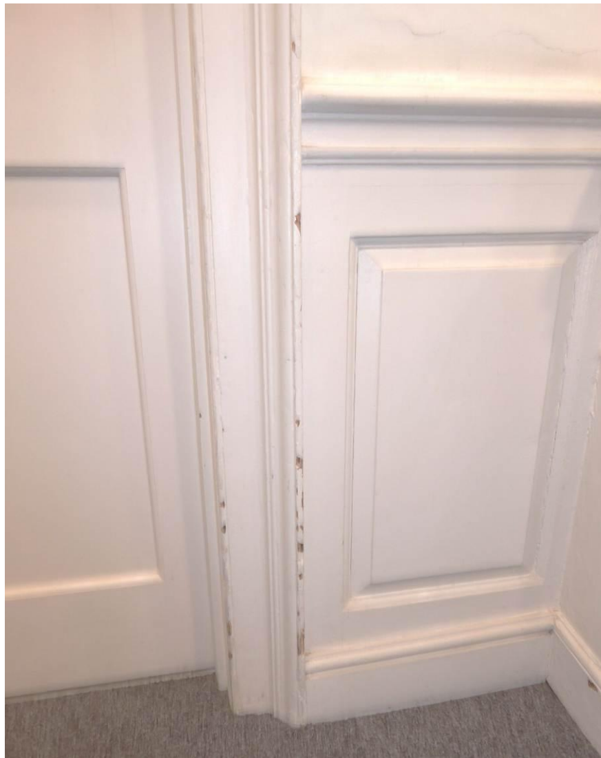
Fig 2.2.1: Timber panelling and typical door lining
