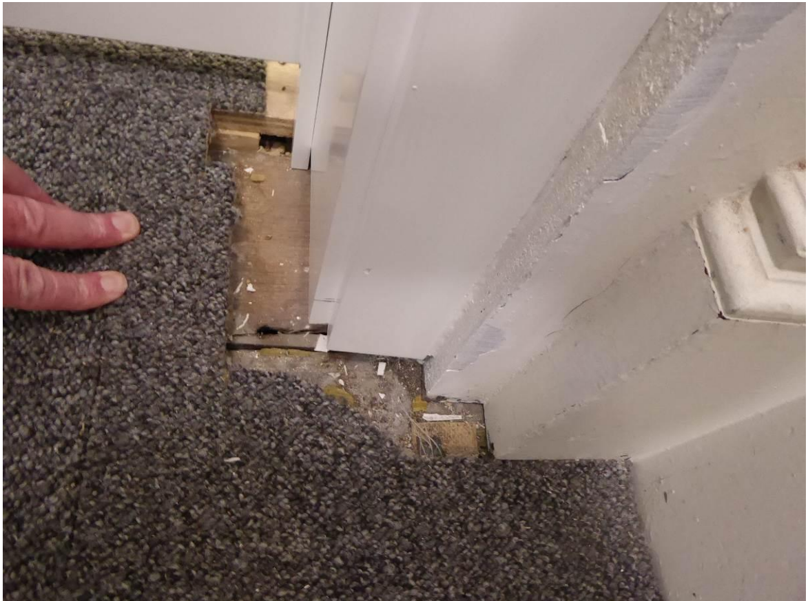
Fig 2.2.3: Widened door opening and lining change
