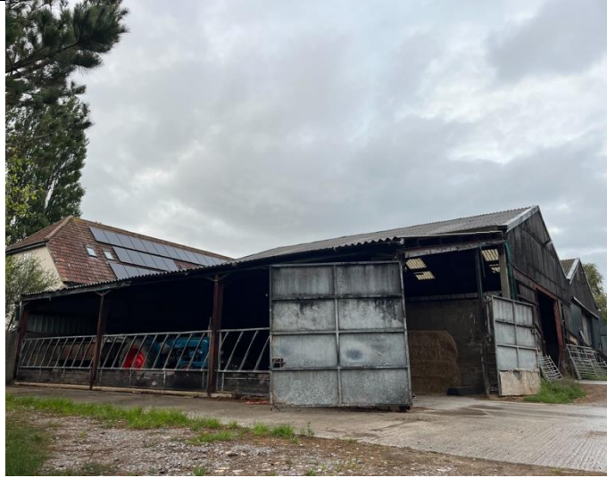
B1 External: south and Western elevation of B1
