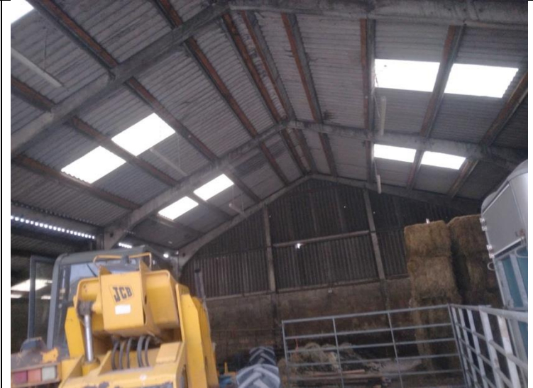
B1 Internal: Western section of B1
