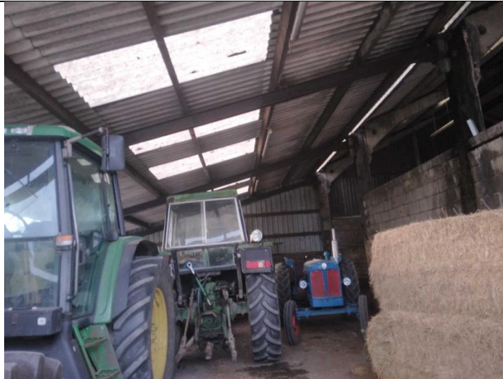
B1 internal: Western section of B1
