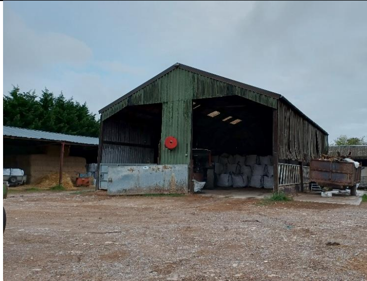
B2 External: north and east elevations of B2
