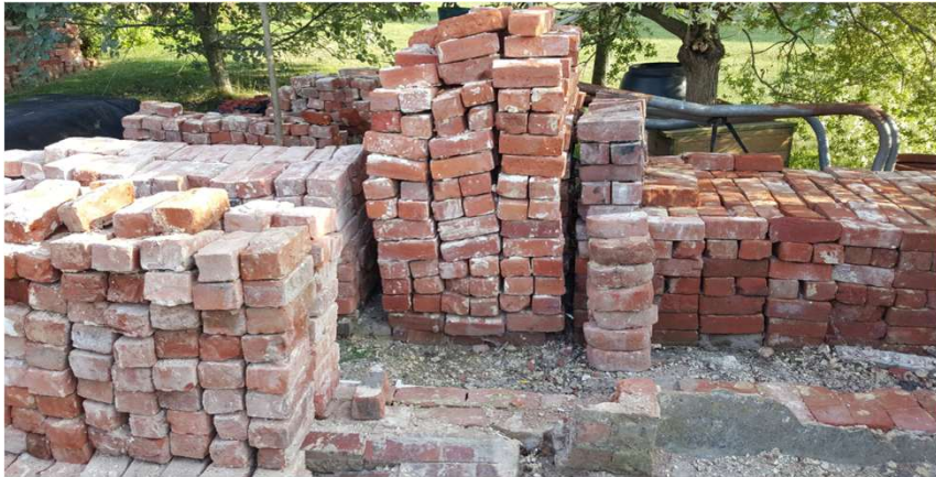
Salvage bricks from collapsed wall
