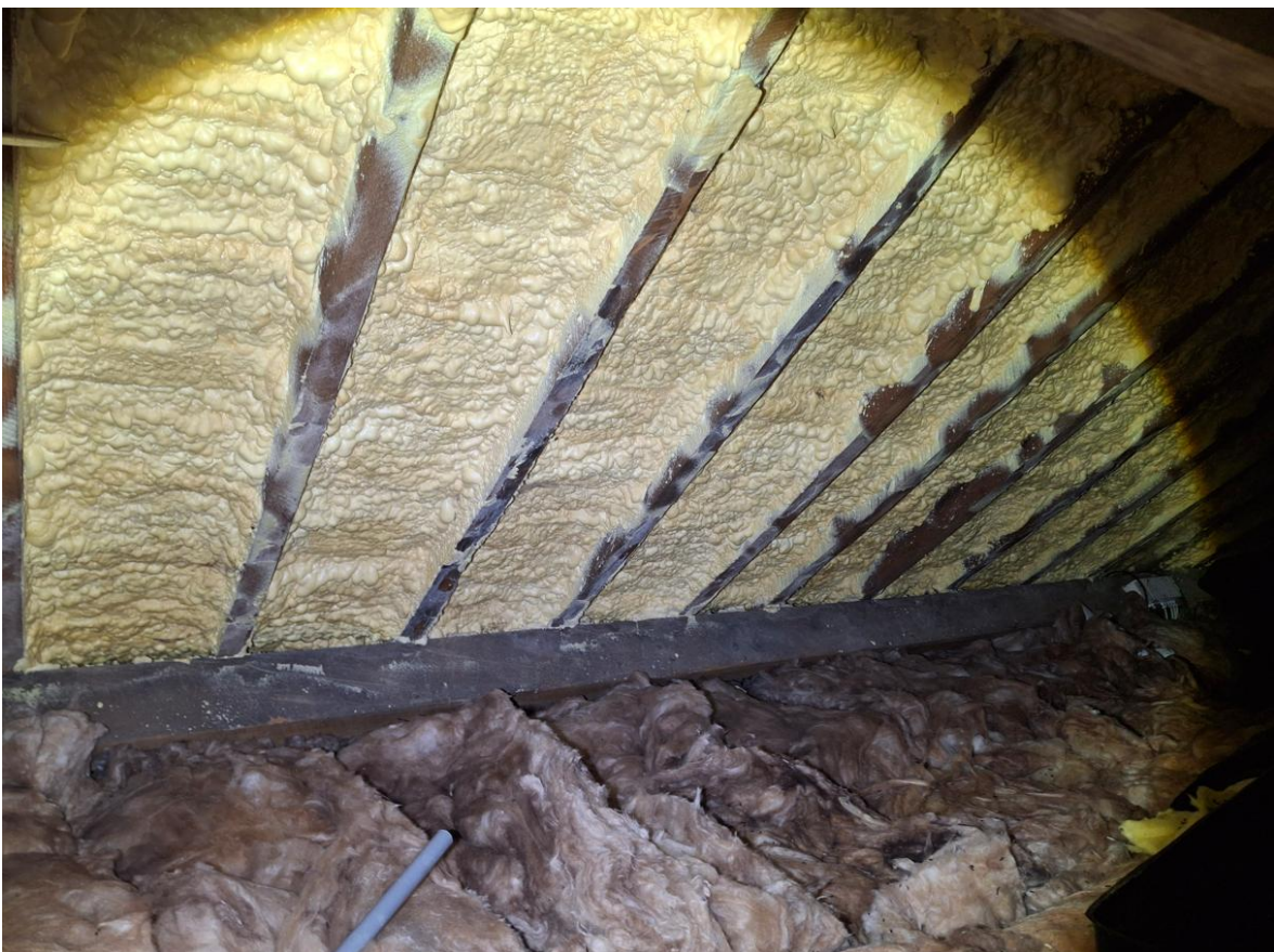
Figure 5: The loft has been sealed with foam insulation
