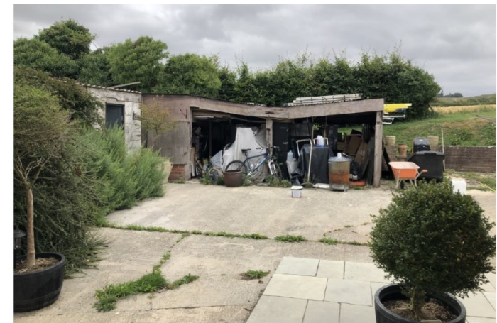
West facing view of the existing brick outbuildings to be replaced with new oak framed building (South east)
