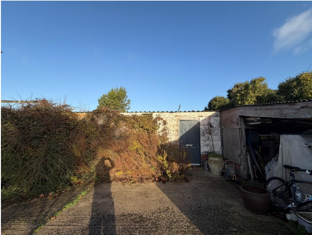
Photograph 5: showing a view of Section 3 of the building
