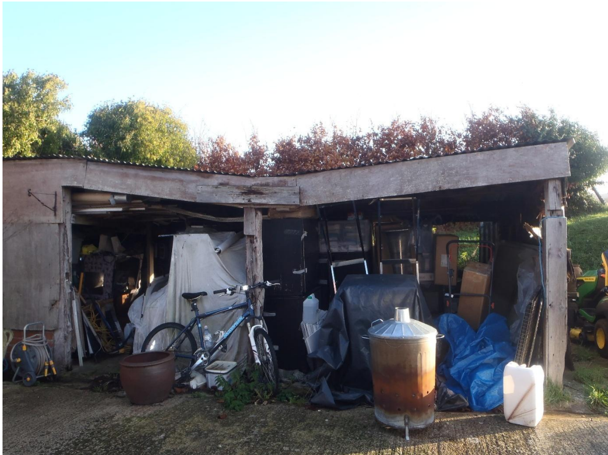
Photograph 3: showing a view of Section 2 of the building
