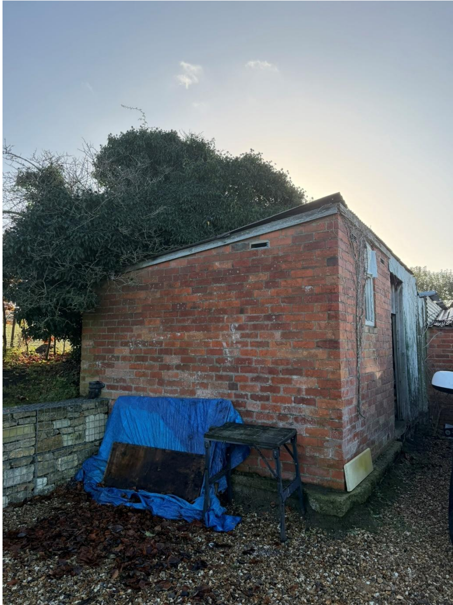
Photograph 2: showing a view of Section 1 of the building
