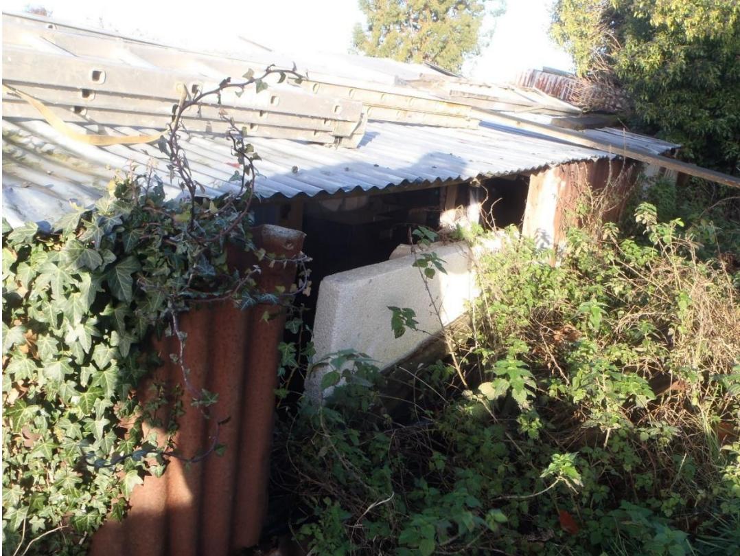
Photograph 4: showing a view of the rear of Section 2 of the building
