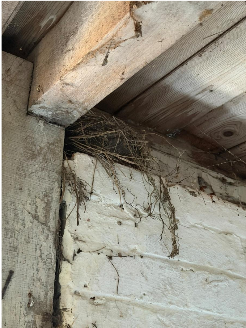
Photograph 8: showing a bird's nest within Section 1 the target building
