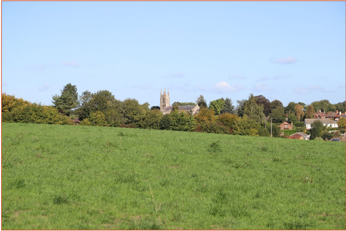
Plate 7 North west facing shot of the upper tower and roof of Christ church (105mm)
