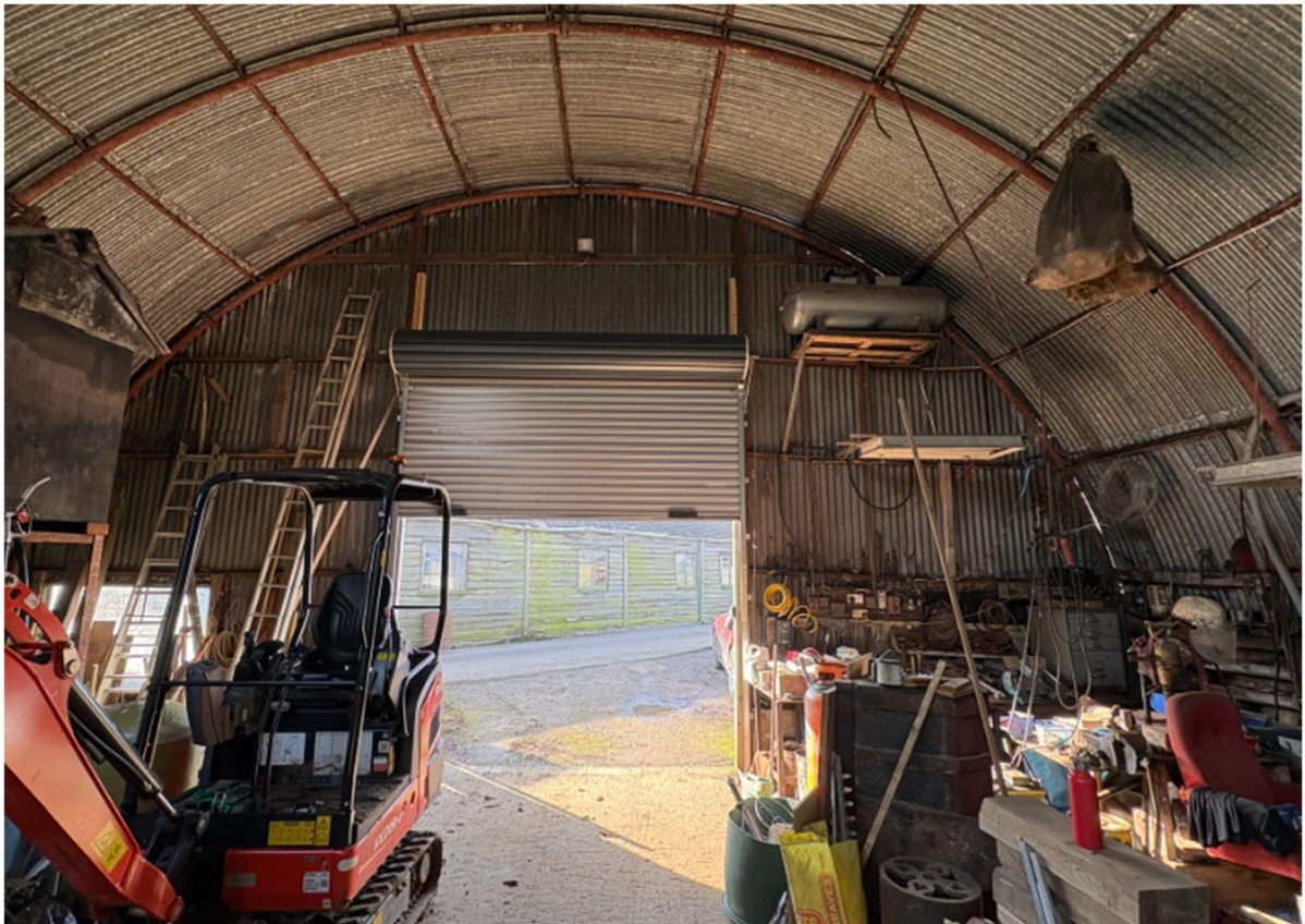
Figure 4. View looking towards main entrance roller shutter door.
