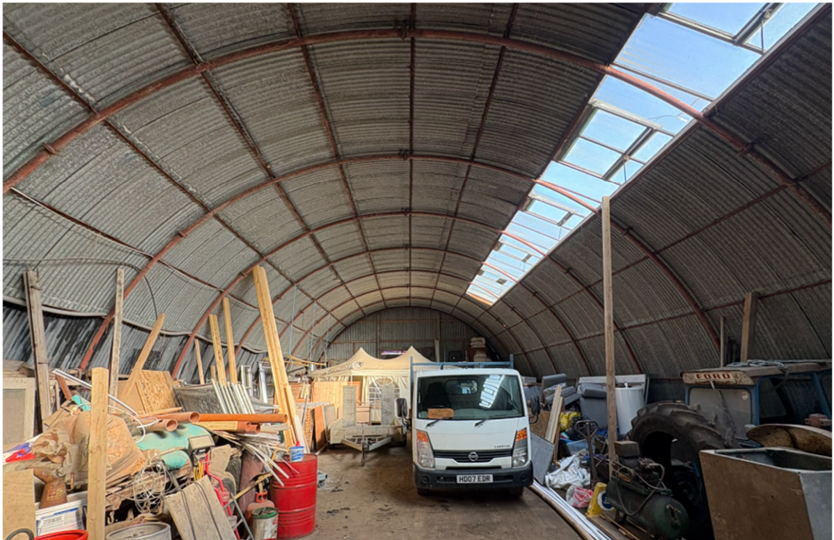
Figure 1. Typical internal view of Building 1.
