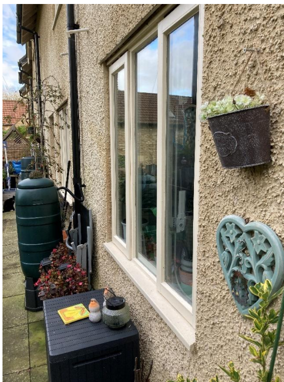
Figure 6: Rear elevation for 3 Smiths Yard, with 4 and 5 visible in the background
