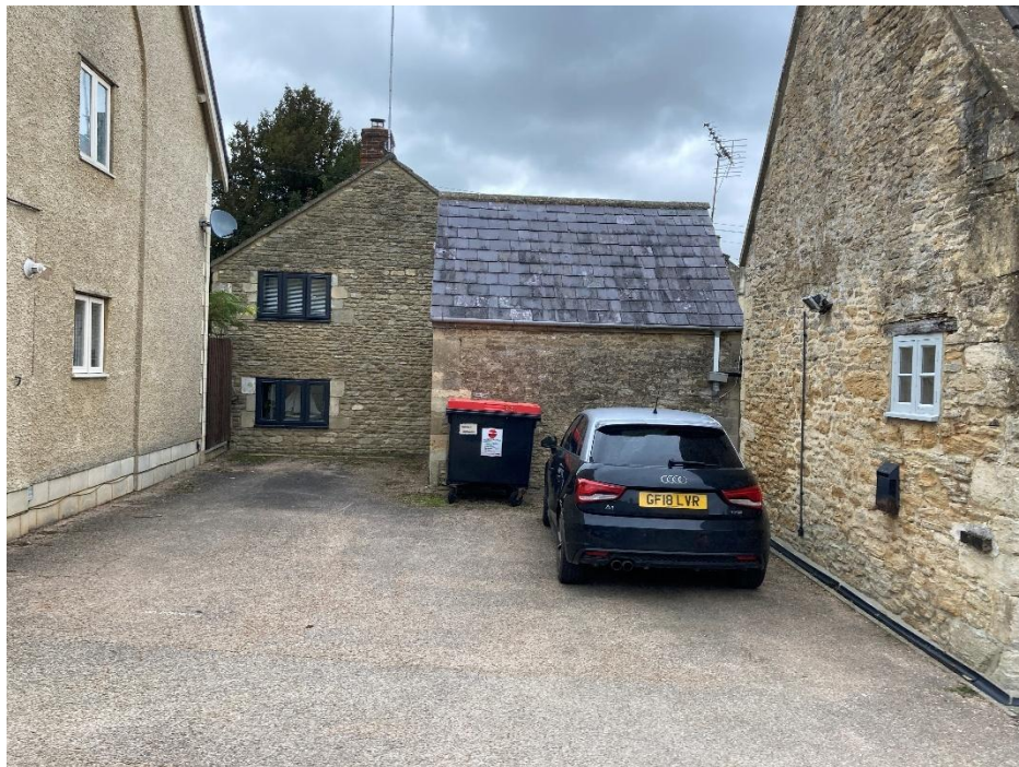
Figure 7: Side elevation of 6 Smiths Yard on left, rear elevation of 51 and 53 High Street on right
