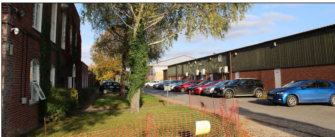
Photo 7. Car parking front of (south-east side) of Portway House
