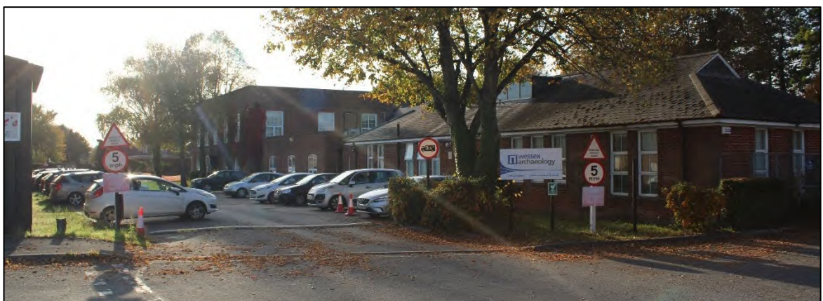
Photo 1. Portway House viewed from the east, showing the Sick Quarters/Infirmary (also known as the Medical Block) in the foreground
