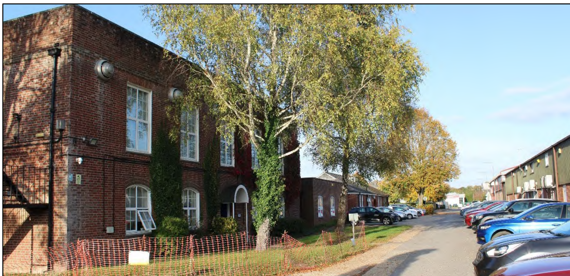
Photo 2. Portway House viewed from the south, showing the Army Cooperation School Building in the foreground
