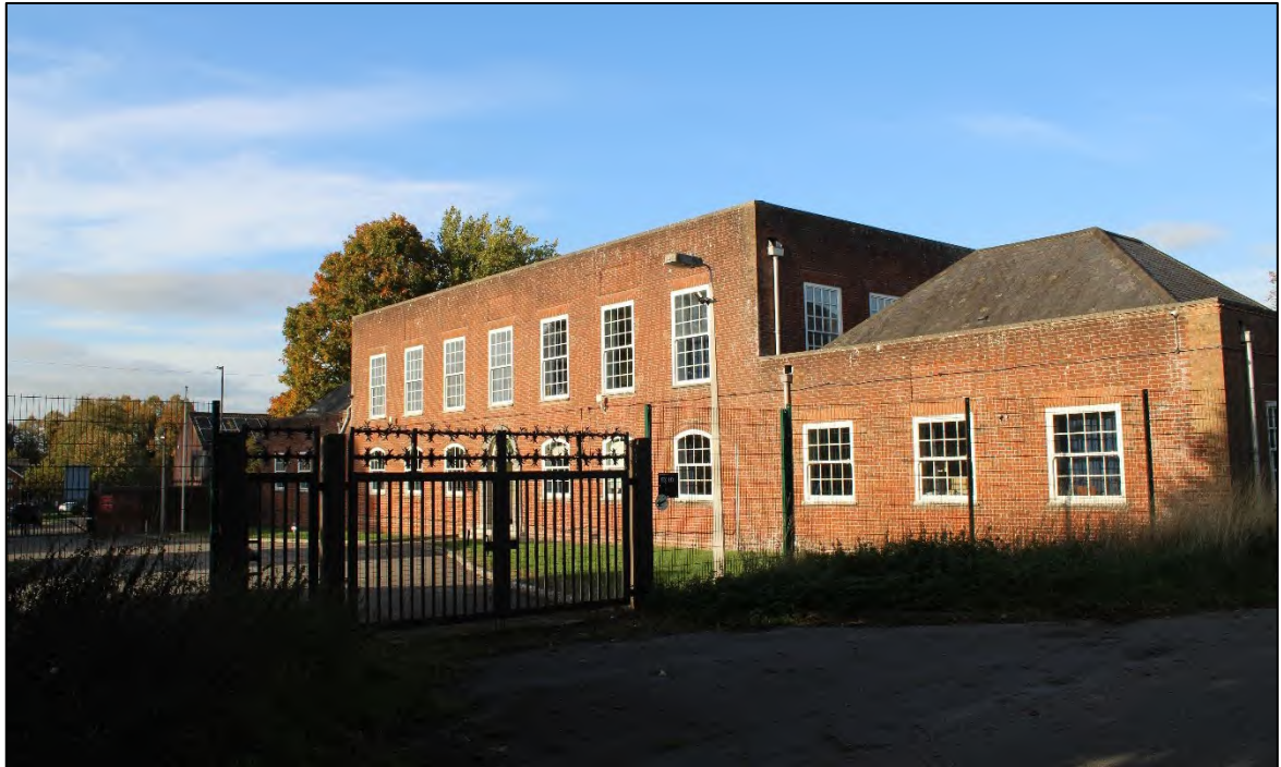
Photo 15 Grade II listed former Station Headquarters viewed from the south (from Lancaster Road)
