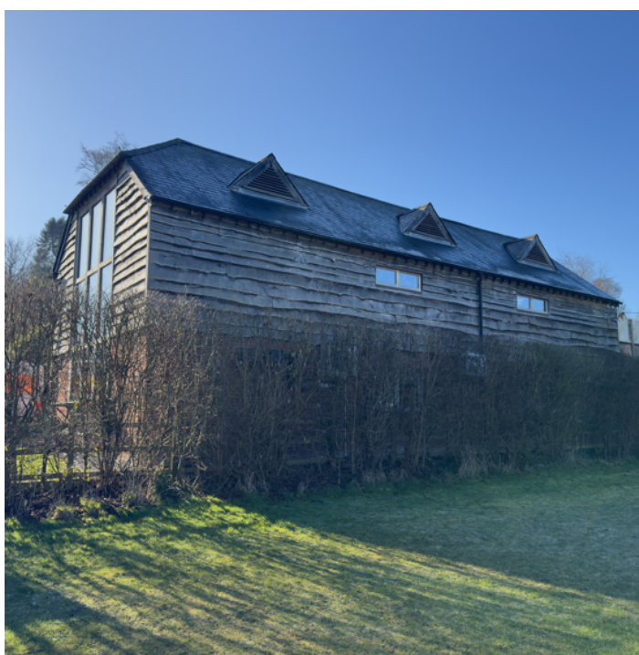
Figure 3 - The northern elevation also showing hazel hedgerow
