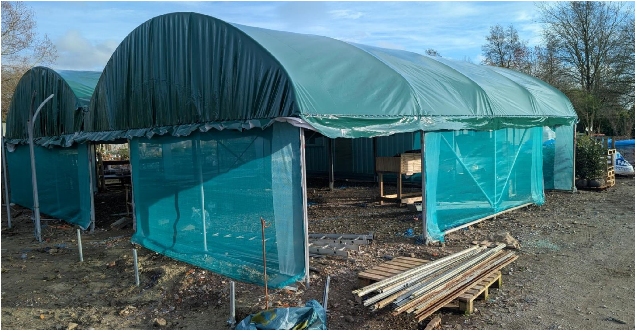
Photo 3: Double Polytunnel A. Construction nearing completion as the date of photograph (14th December 2025)
