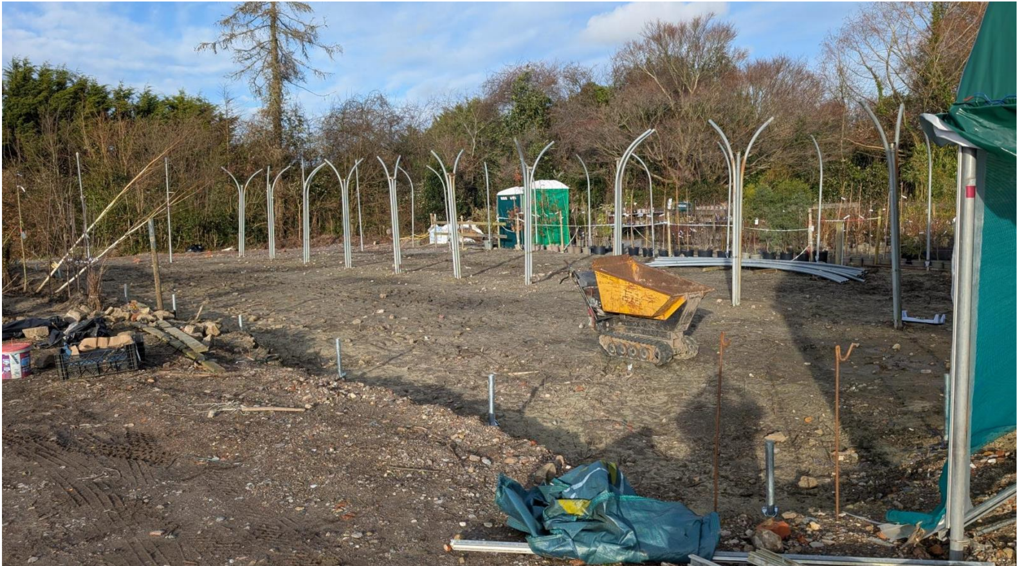
Photo 2: The second Double Polytunnel B currently under construction (NB. date of photograph 14th December 2025)
