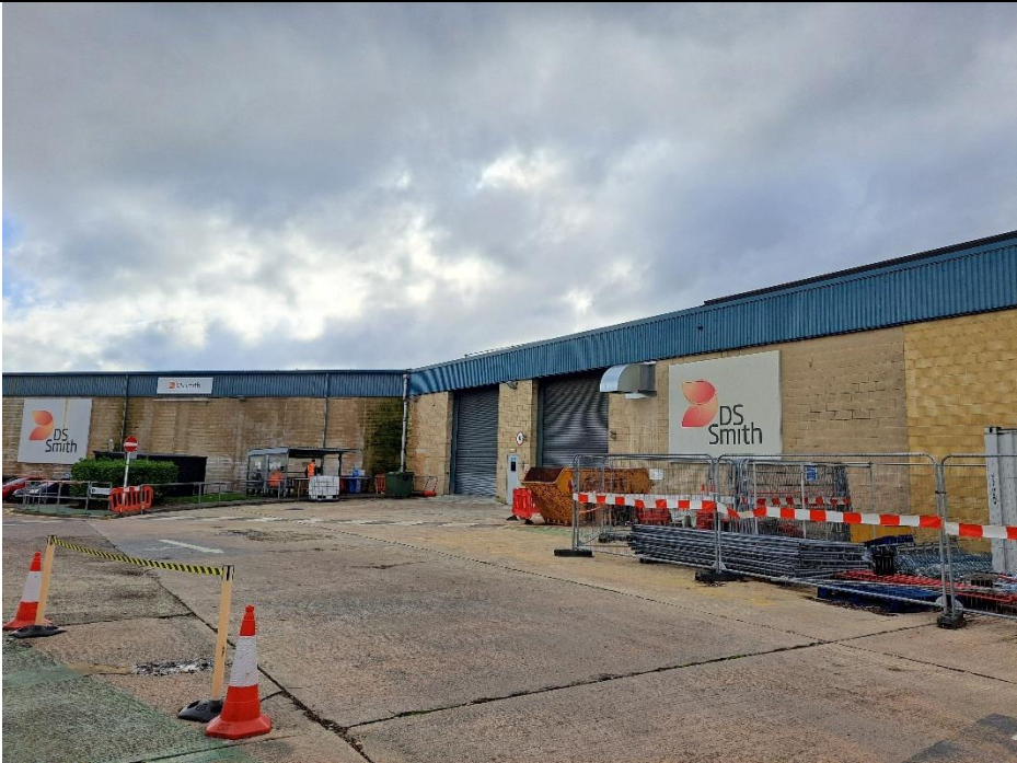
North-east view of external elevation.
