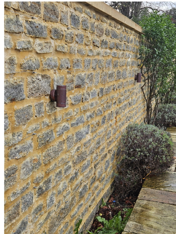
D - View of new wall constructed from Cotswold rubble stone laid in courses
