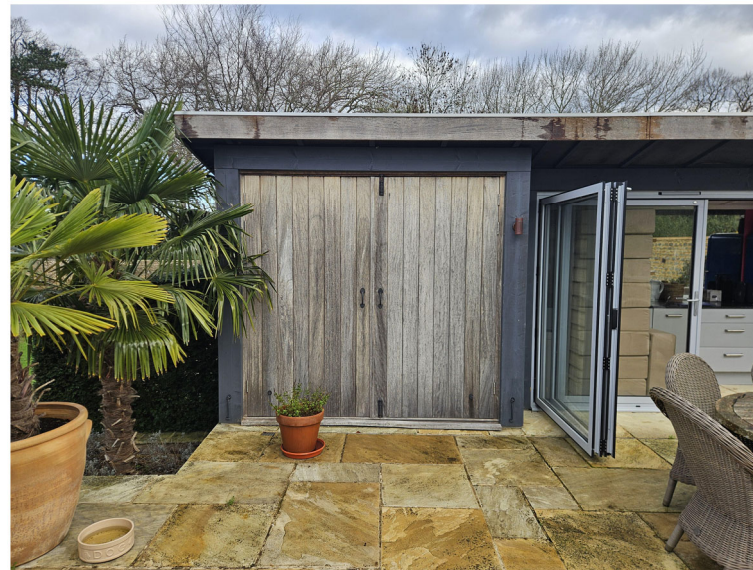
F - View of outbuilding storage area - Store doors in bevel-edged, close-boarded iroko Panels
