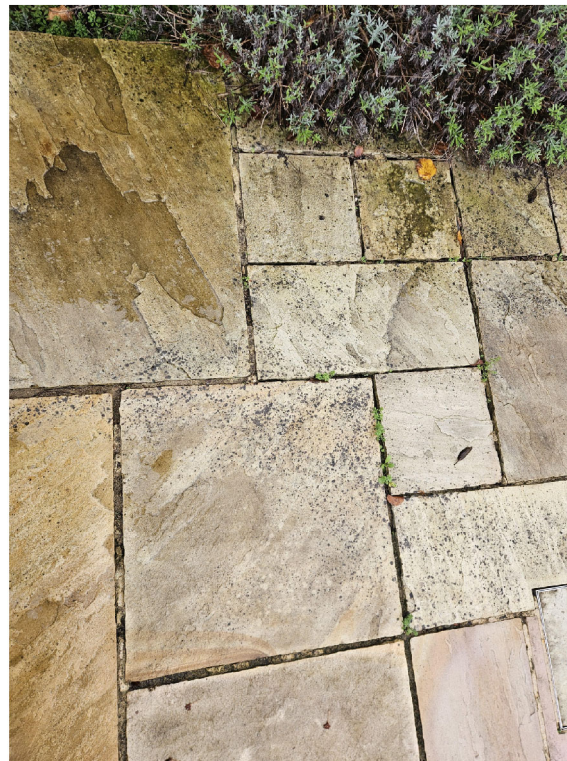
C - View of new natural stone paving to swimming pool area
