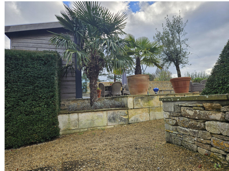
G - View of side of new outbuilding and boundary - Iroko weatherboard, over ashlar wall with stone capping
