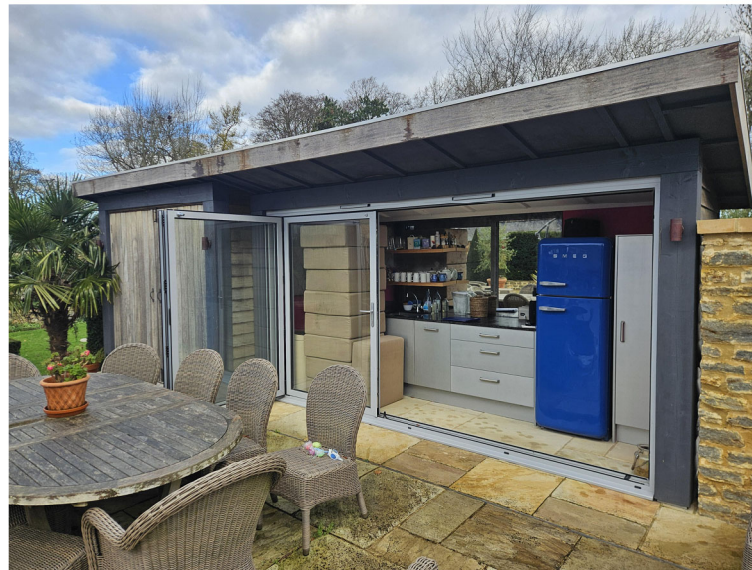
E - View of outbuilding, housing outdoor kitchen and storage - Kitchen doors in aluminium frames (RAL 9006)
