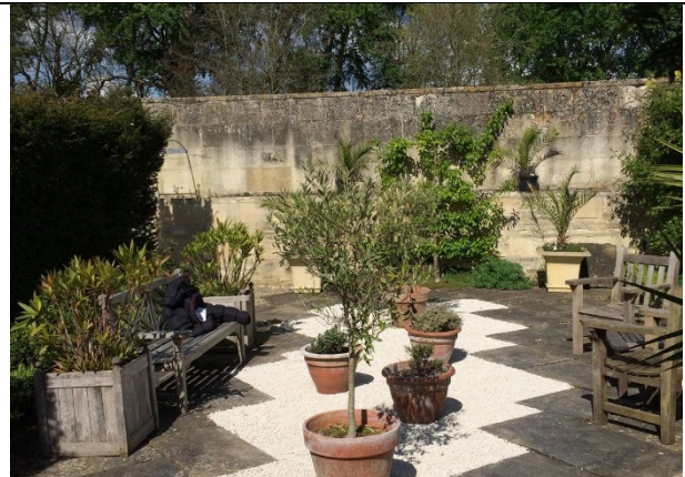
View of Demolished wall to boundary of side garden
