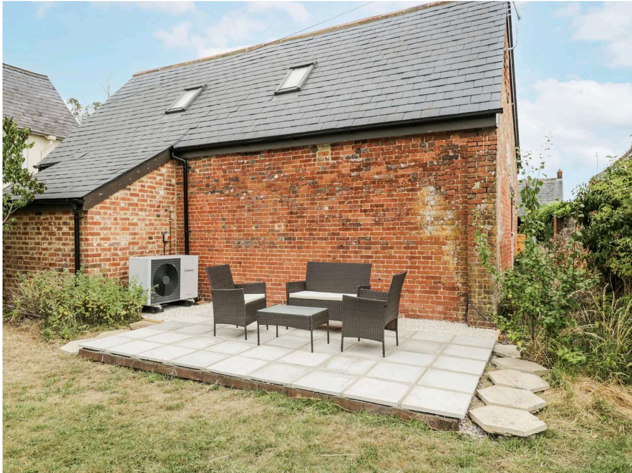
Fig 2. The Coach House from the rear showing rear amenity space. New rooflights are the only addition to the external fabric.
