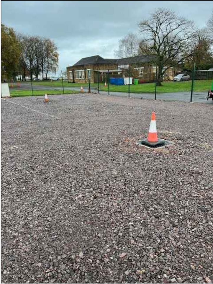
New Hardstanding consisting of: - Non-woven membrane - 6 inches of limestone quarried - 2 inches of Type 1 CF5 Capping quarried
