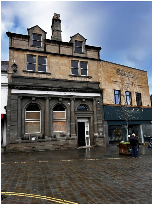
Image 2: Main elevation to application building fronting on to Market Place (newly refurbished 1 Market Place to the right of the application building)
