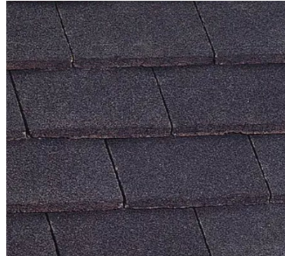
Roof – Plain concrete tiles to match existing
