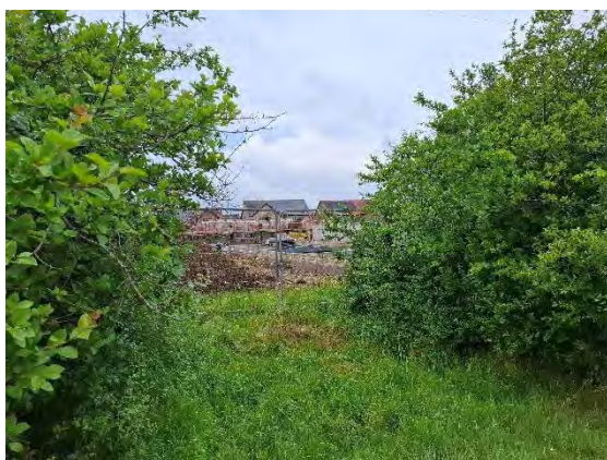
Photograph 17: View of construction site to the north through hedgerow
