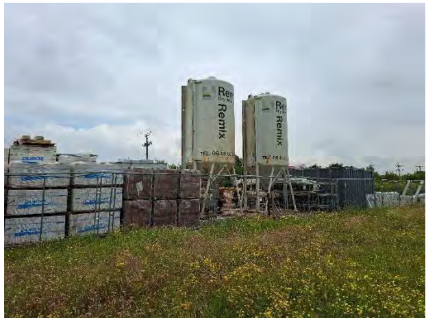
Photograph 16: Construction storage area within the north of the site
