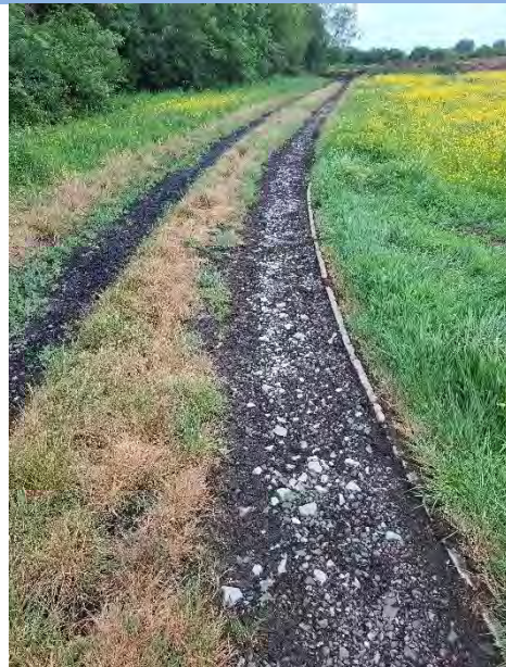
Photograph 4: Gravel track with concrete edging
