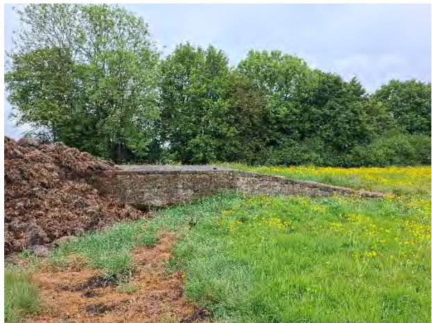
Photograph 10: Concrete ramp next to stockpile
