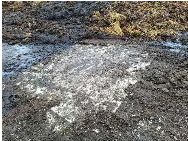
Photograph 8: Concrete slab next to stockpile
