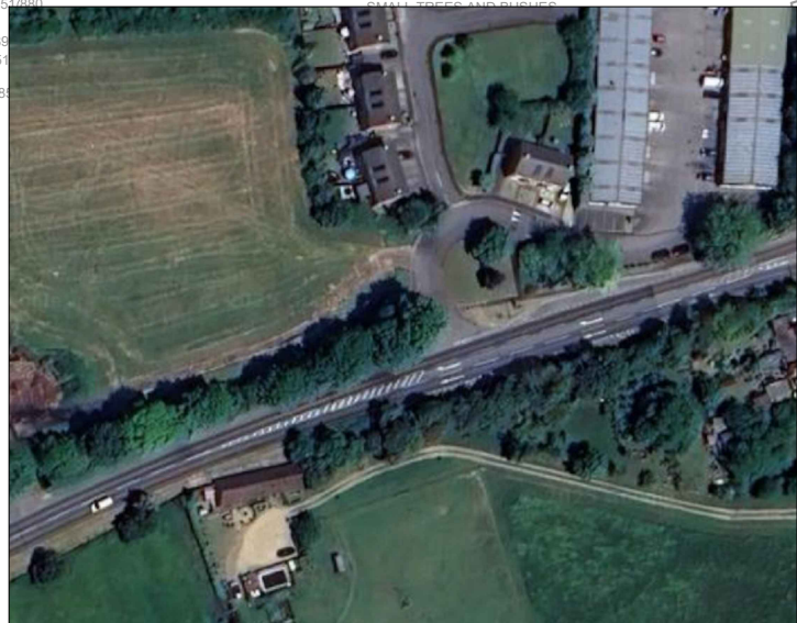
NORTH SOUTH AERIAL VIEW
