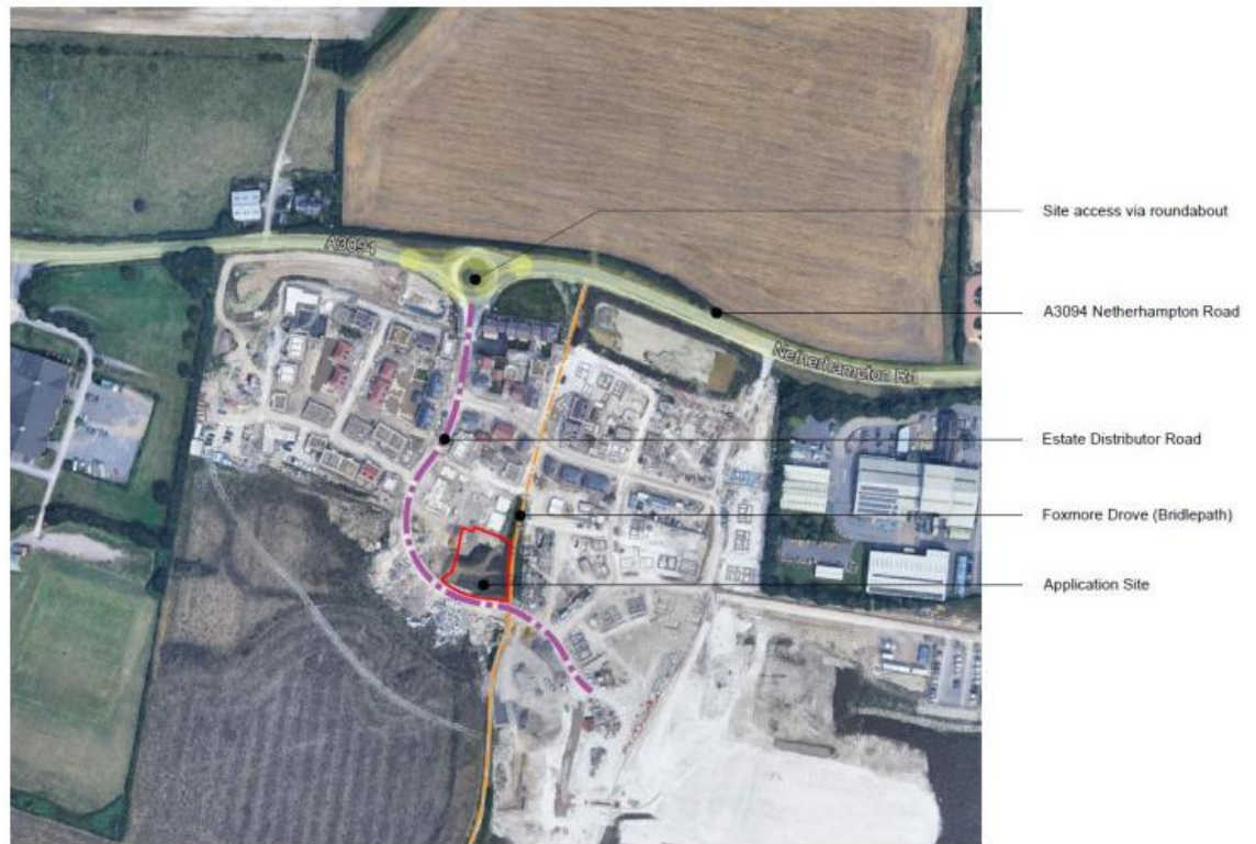
Figure 1. Aerial view of retail plot location at Wilton Gate
