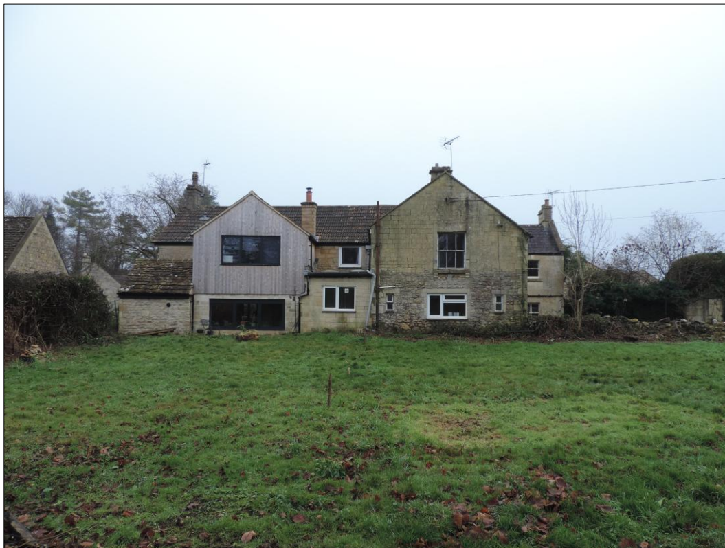
Photo 1 The Project Site, facing east towards the rear / side elevations of nos. 33 & 39 Winsley non-designated heritage assets.
