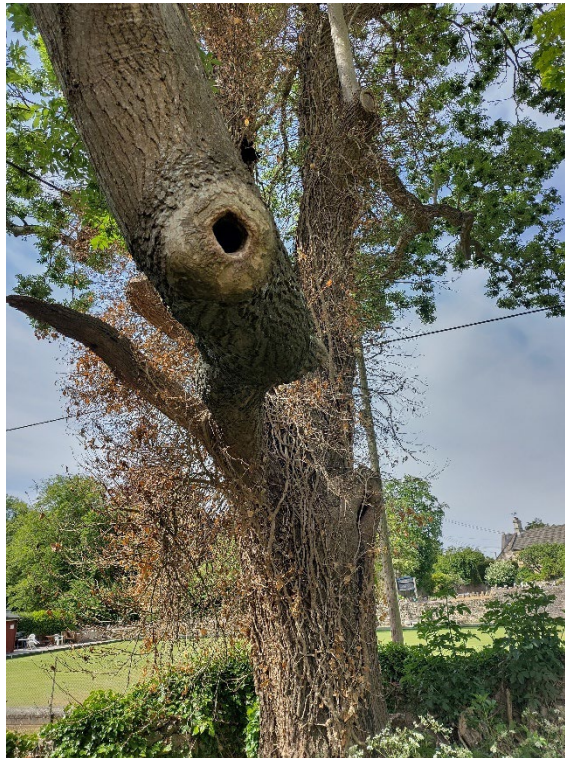
Photograph 3. T8 with rot holes suitable to support roosting bats
