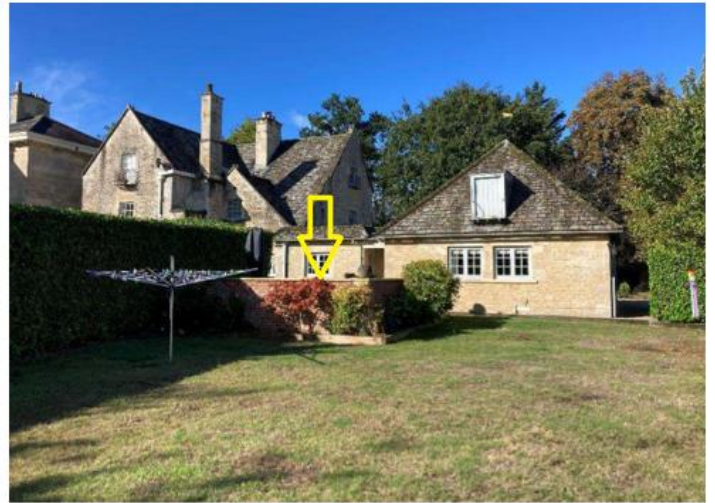
View of the rear, (east) elevation of Butlers Quarters, looking south-west.
