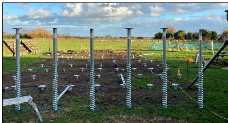
Picture 2: An example of a ground screw system
