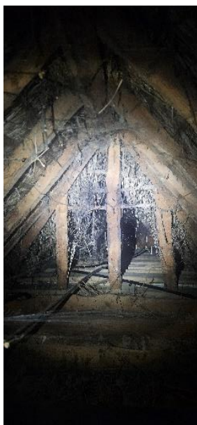
Photo 11: Looking west in the cottage void.
