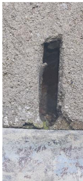
Photo 10: Close up of the gap in the brickwork/render on the southern elevation of the cottage.
