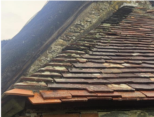
Photo 5: Gaps underneath bonnet tiles and raised main tiles on western elevation of the storeroom.
