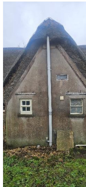
Photo 8: South elevation of the cottage.
