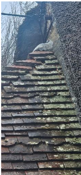
Photo 5: Gaps underneath bonnet tiles and raised main tiles on western elevation of the storeroom.
