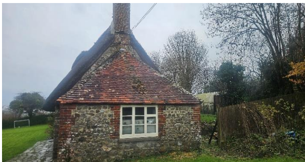
Photo 3: Western elevation of the storeroom.
