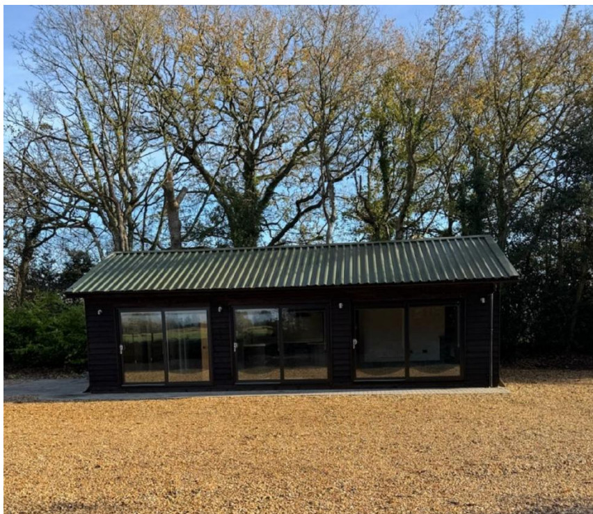
Above – views of completed dwelling
