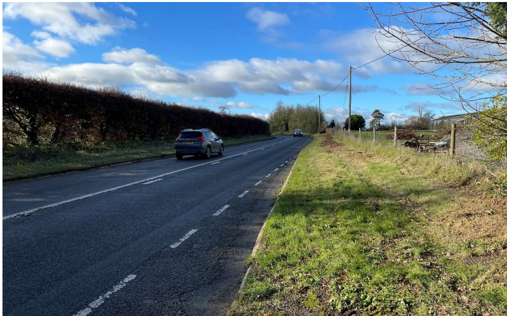
Figure 3: Visibility Splay – view west along Westbrook Road
