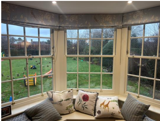
Existing double glazed sash windows below
