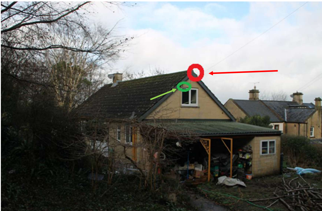
Figure 2: showing bat access/egress location
